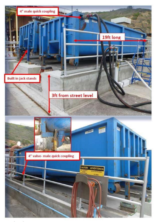
Revised: April 29, 2016 OCA Document No. 1277089 The containers at NCWRP shall not exceed 19 feet in length and not exceed 7 feet in height. The NCWRP wet sewage scum container fill hatch shall be on the left rear (drivers) side and top of the container which will accommodate the NCWRP fill line to fill the container. The container shall have a bottom decant line with a valve on the bottom of the container used for decanting as described above. **See photo below**.
