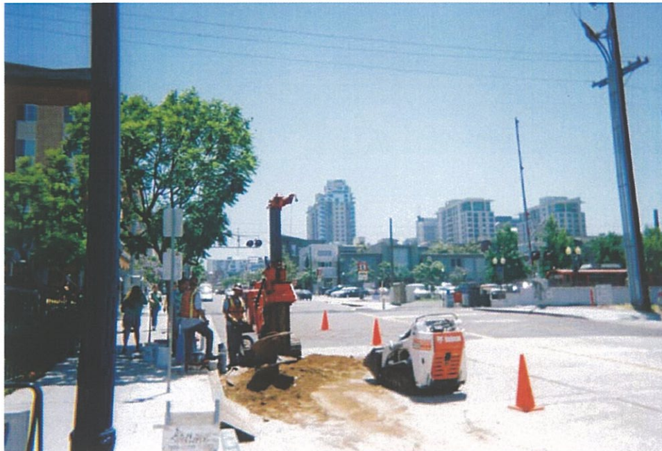
MINI BUCKET AUGER RIG USED TO DRILL LARGE DIAMETER BORINGS.
