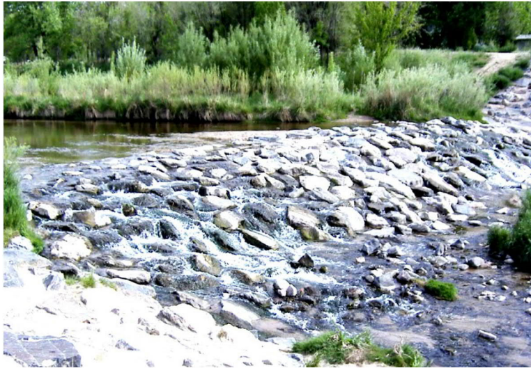
Figure 7-18. Example of Sloping Grouted Boulder Drop Structure
