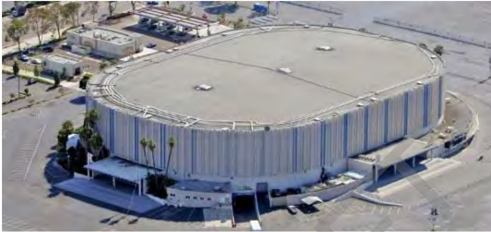
Aerial View of Exterior Existing Precast Concrete Double Tee Exterior at Pechanga Arena
