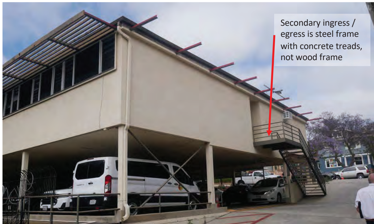
Large steel frames and girders with concrete pilings are visible under the parking area. This structure is not representative of wood Post & Beam architectural style.
