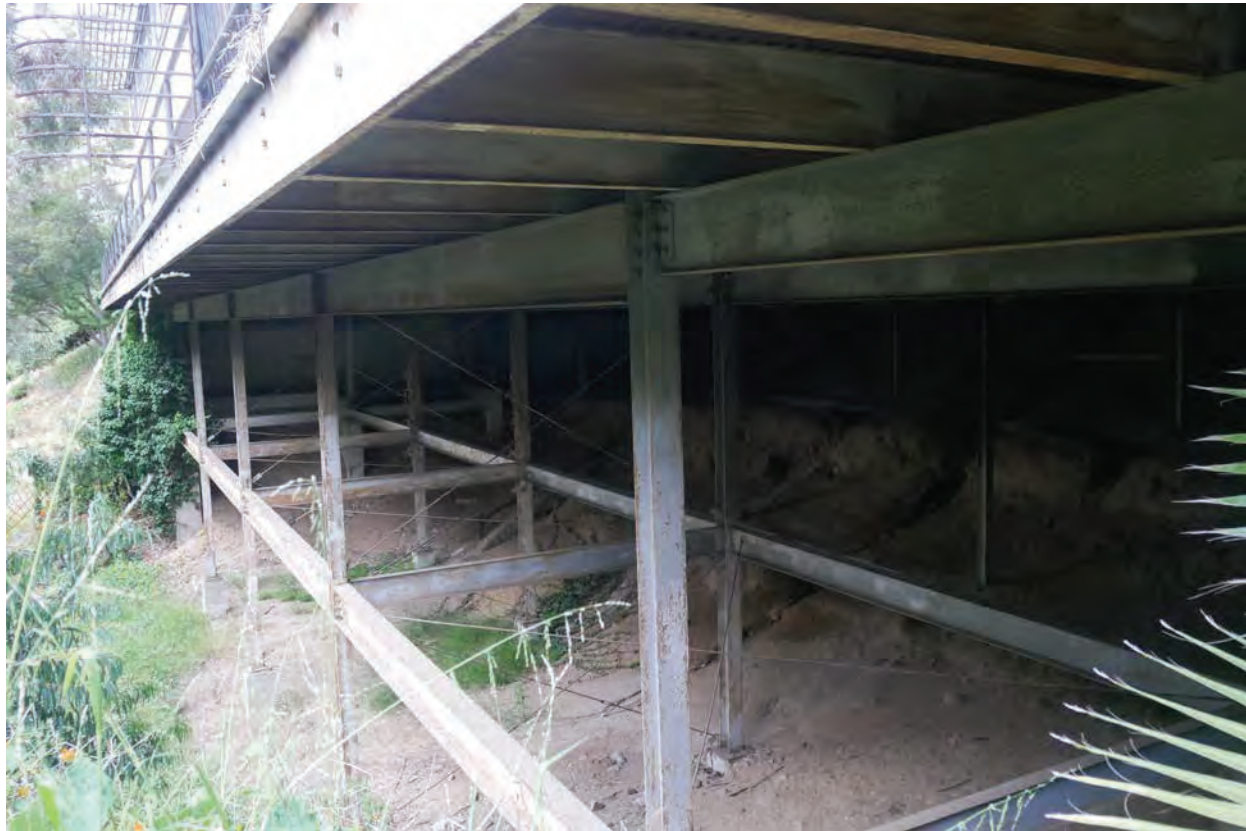
Large steel frames and girders with concrete pilings are visible under the parking area. This structure is not representative of wood Post & Beam architectural style.
