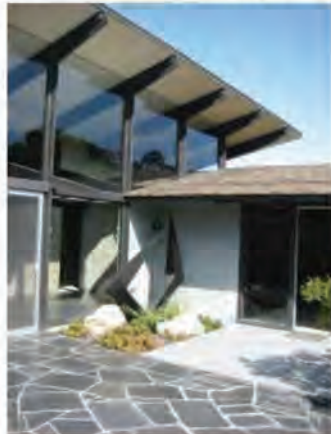
The Mills residence in La Jolla, designed by Dale Naegle in 1957. Note the scissor rafters in the entry foyer and the dramatic full-height glass. The arrangement of the floor plan around a central courtyard and the continuous interior/exterior flooring add to the strong outdoor connection.
