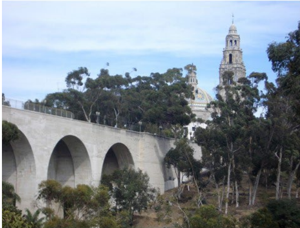
Cabrillo Bridge and Balboa Park
