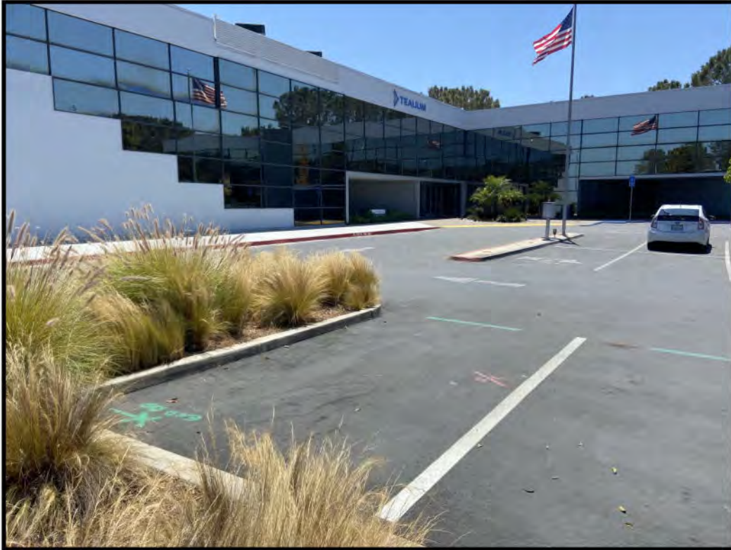
1. Existing building at 11095 Torreyana Road.
