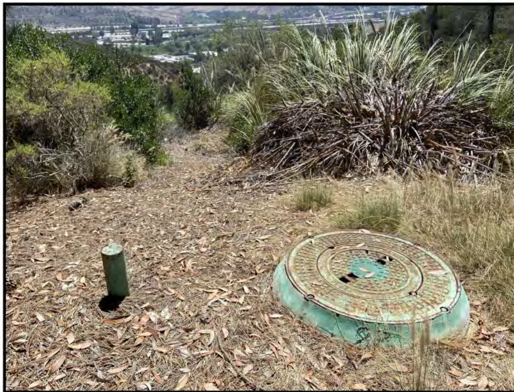
10. Southern sewer easement and view toward east.
