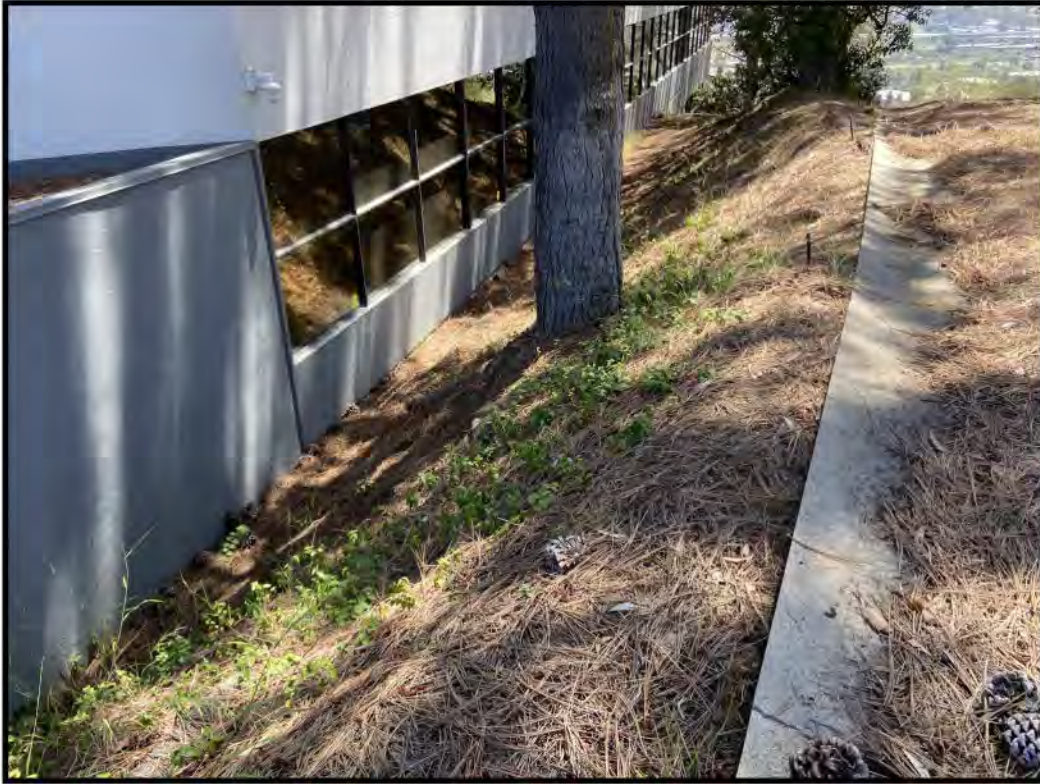
9. Southern edge of 11085 and Site with Torrey pines planted along building.
