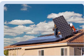
Installation of a solar energy system
