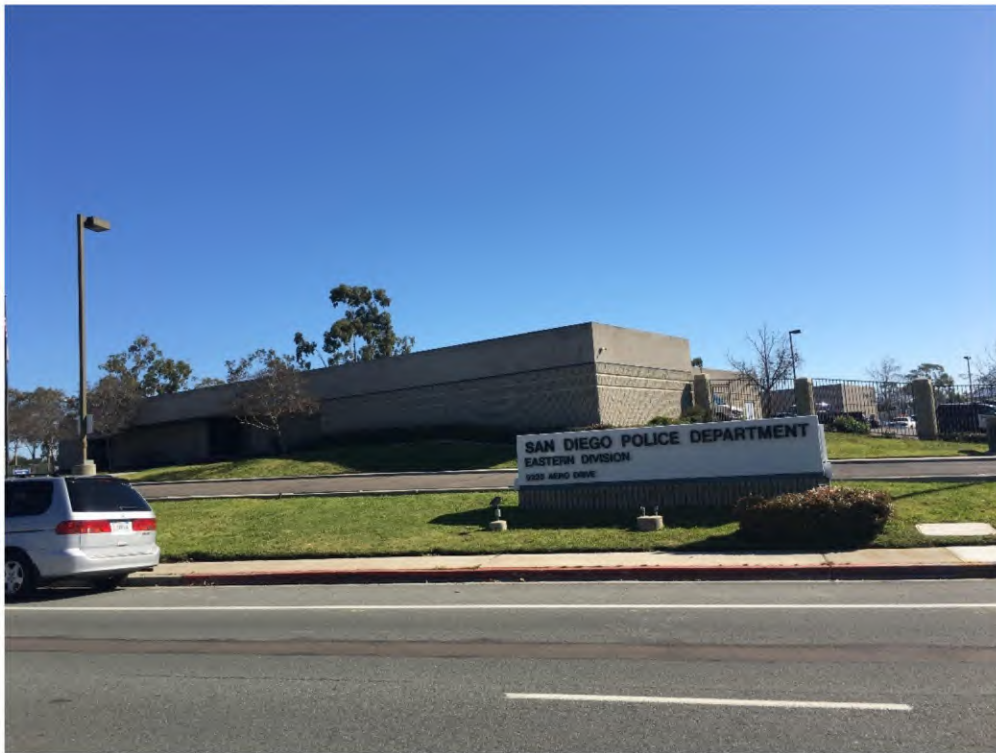
View of San Diego Police Station located on the southeast portion of the Site.
