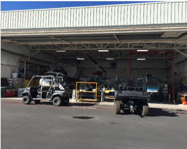
View of San Diego City Police Air Unit Hangar in the west portion of the Site.
