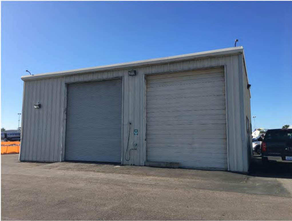
View of the shed which historically held a fire truck with a 500 gallon tank for fire suppression located in the central portion of the Site.
