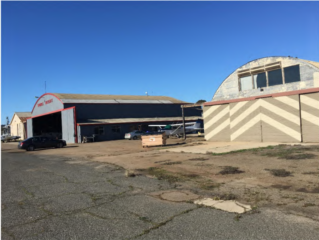
View of Spider's Aircraft Service buildings in the west portion of the Site.
