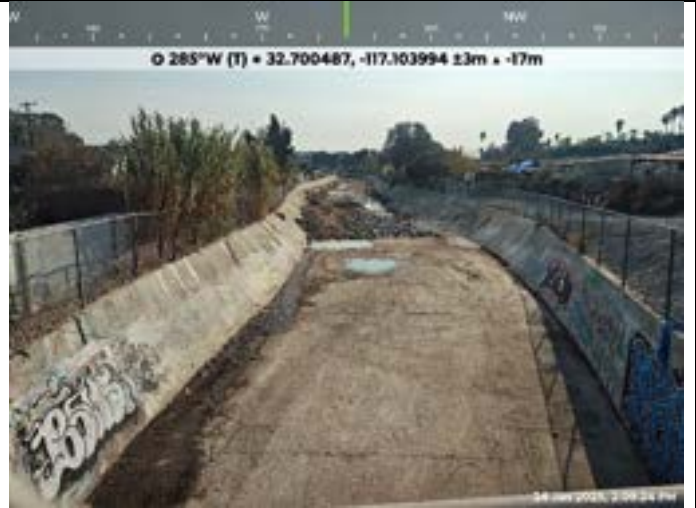
Oceanview 1 Post-Maintenance- Photo 2
