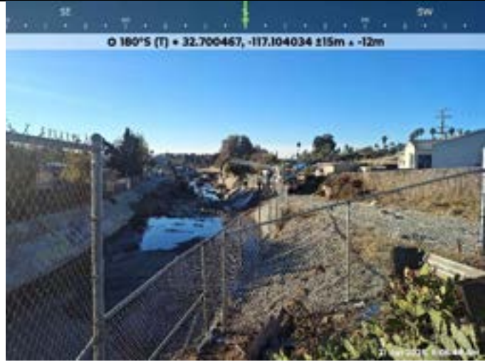
Oceanview 1 Pre-Maintenance- Photo 1
