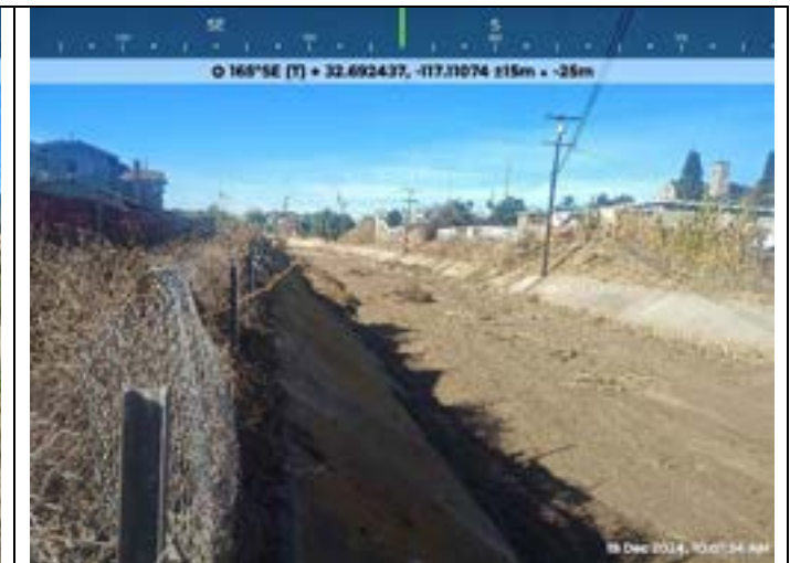
Alpha 1 Post-Maintenance- Photo 2
