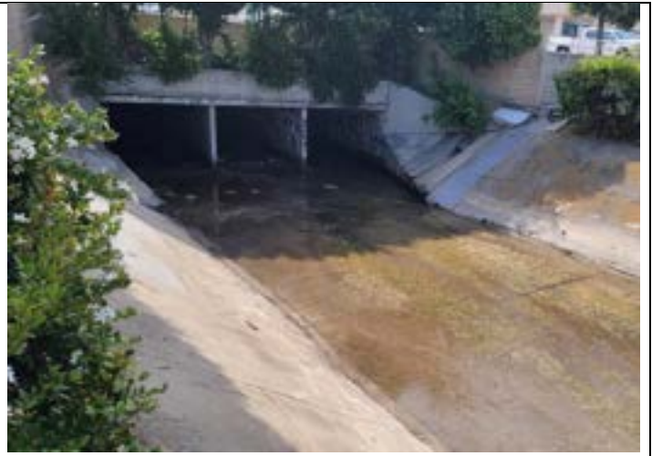
Mission Gorge 2 Post-Maintenance- Photo 2
