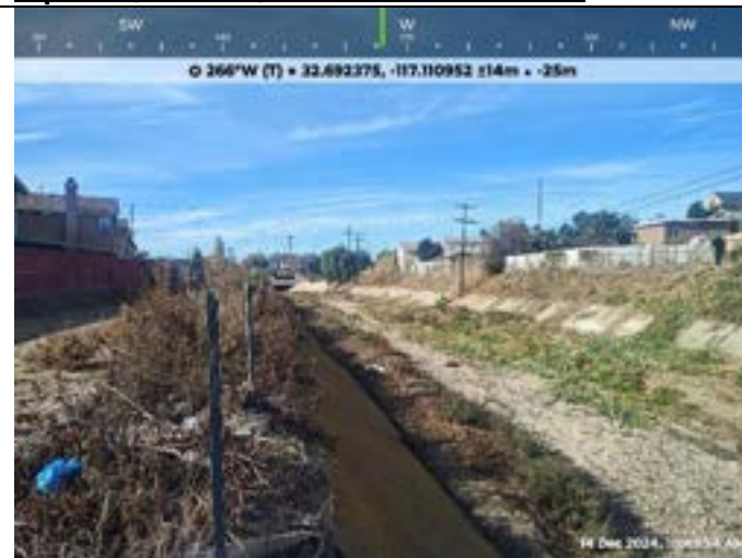
Alpha 1 Pre-Maintenance- Photo 1
