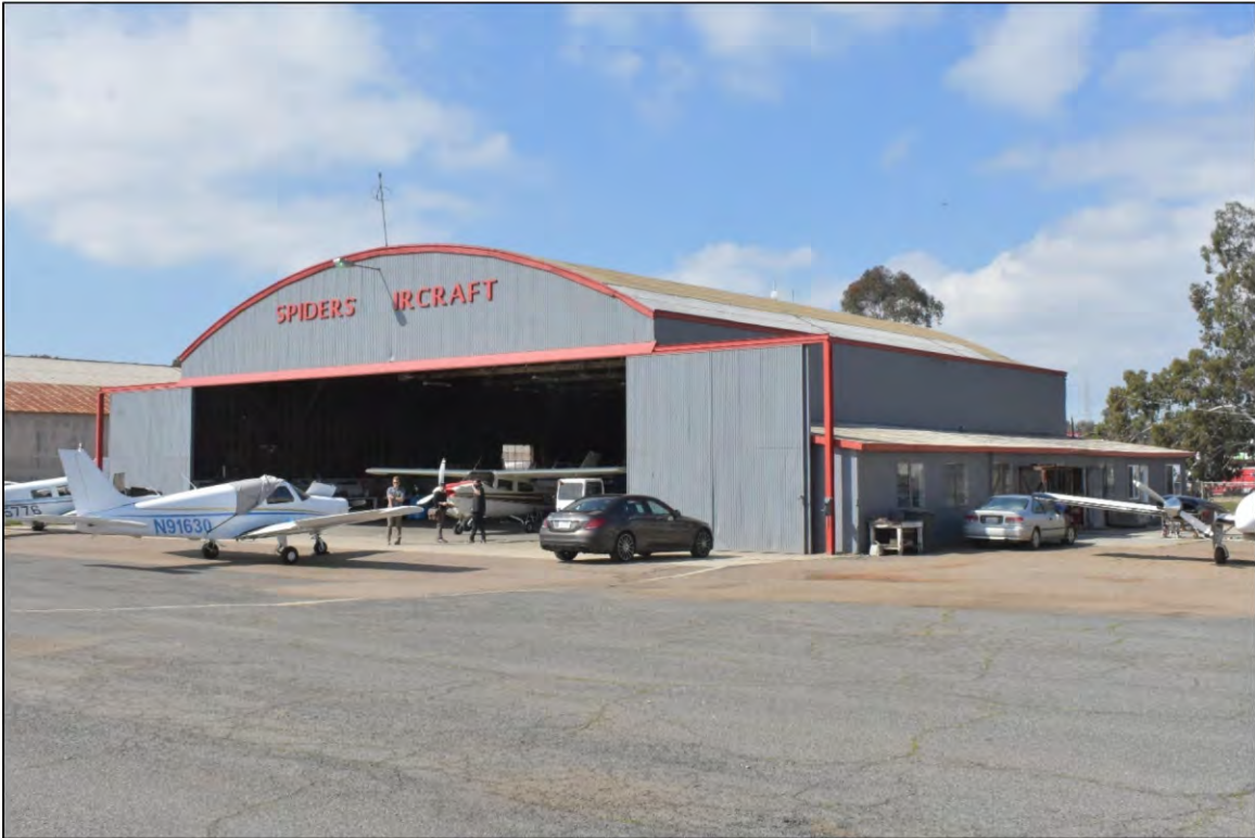
Figure 44: Three-quarter view showing Building 7 east and north elevations.
