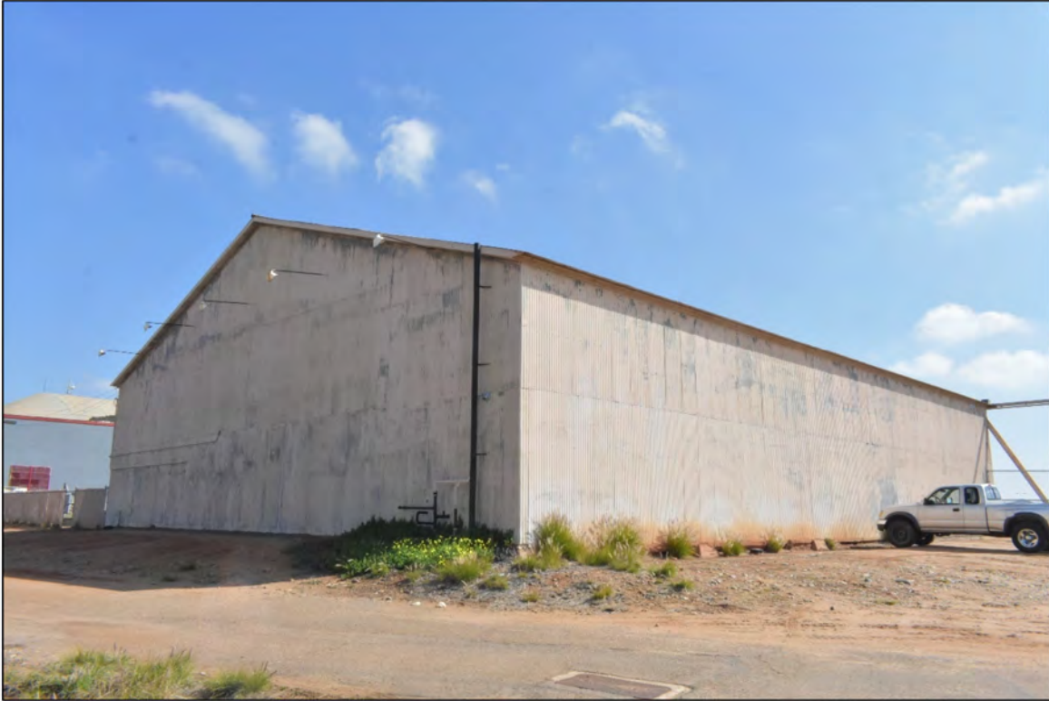
Figure 53: Three-quarter view of the south and west elevations of Building 8.
