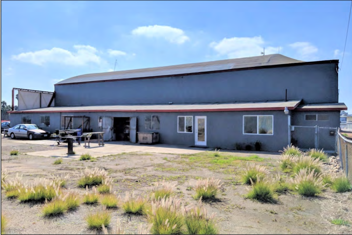
Figure 48: Building 7 North elevation with shed roof addition.
