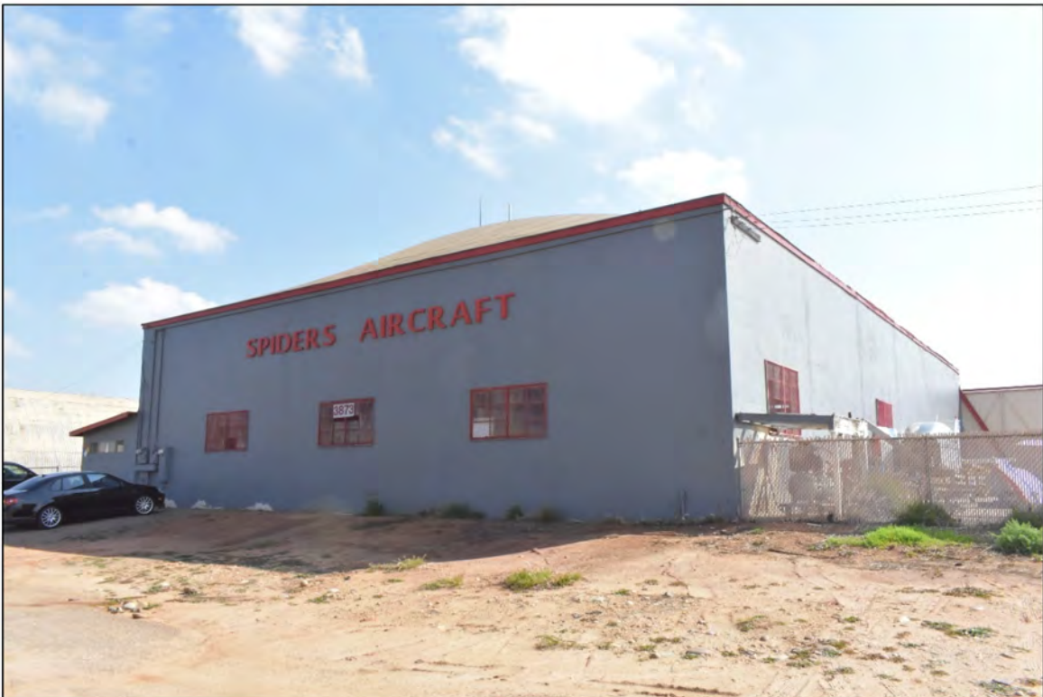
Figure 47: Three-quarter view of Building 7 east and south elevations.
