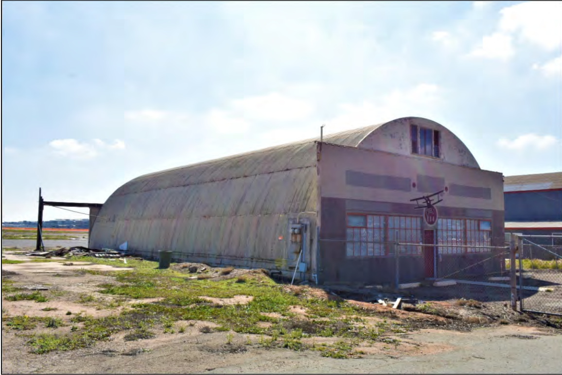
Figure 32: Three-quarter view showing the north and west elevations.
