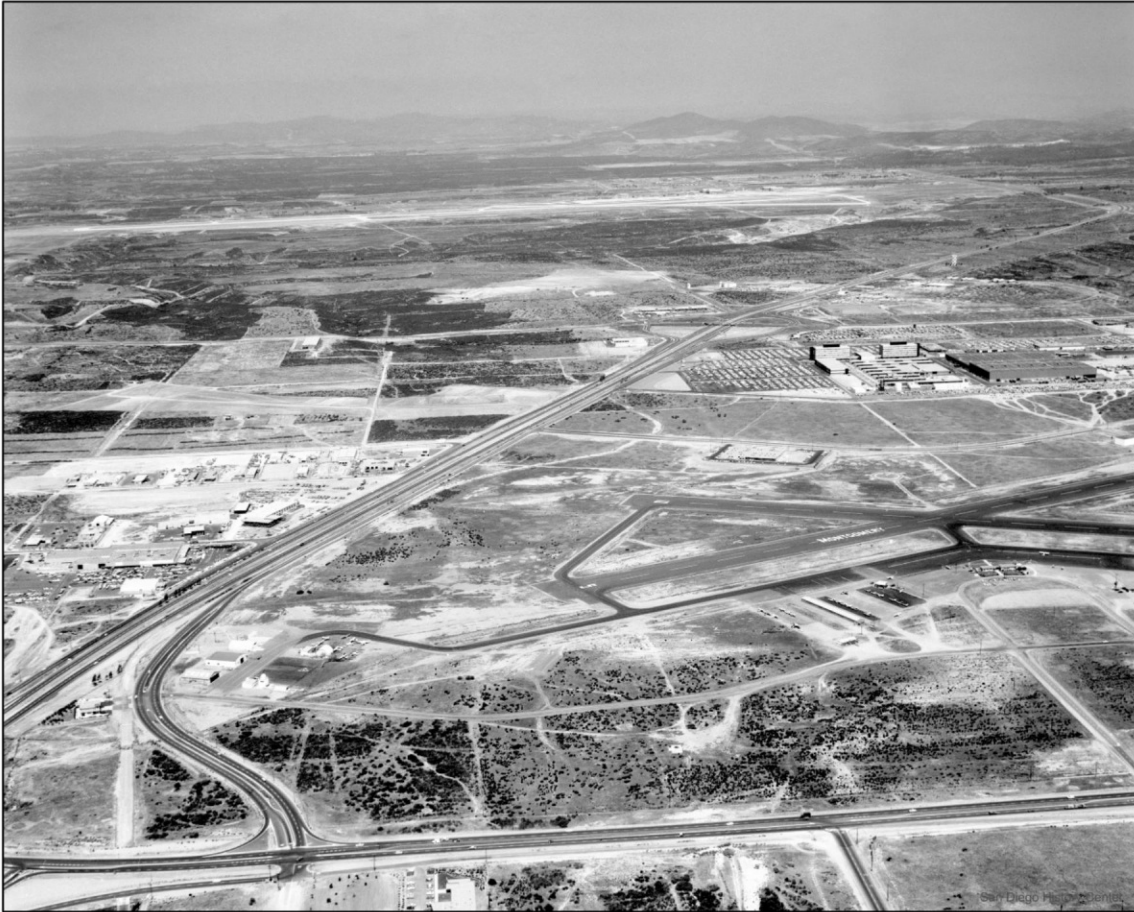
Figure 17: Montgomery Field and Kearny Mesa in 1960. San Diego History Center, 92_18835-2095 Montgomery Field - General Dynamics - aerial - 1960
