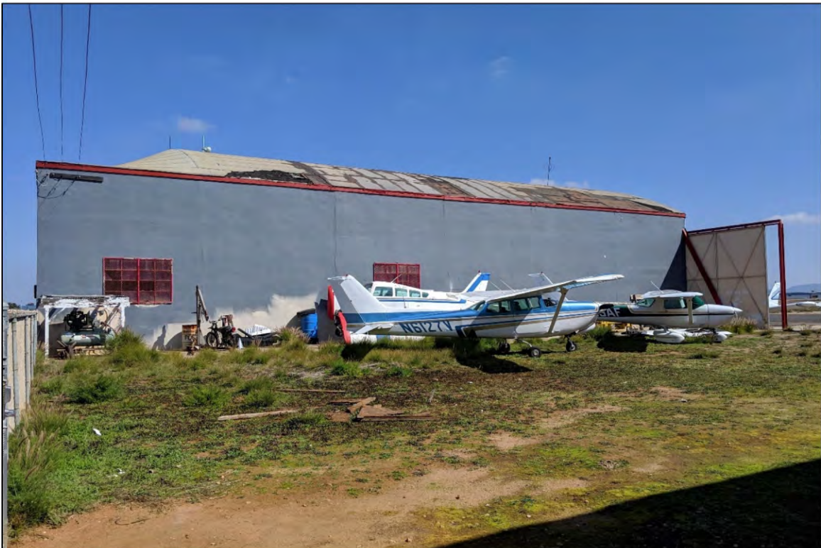
Figure 45: Building 7, South elevation.
