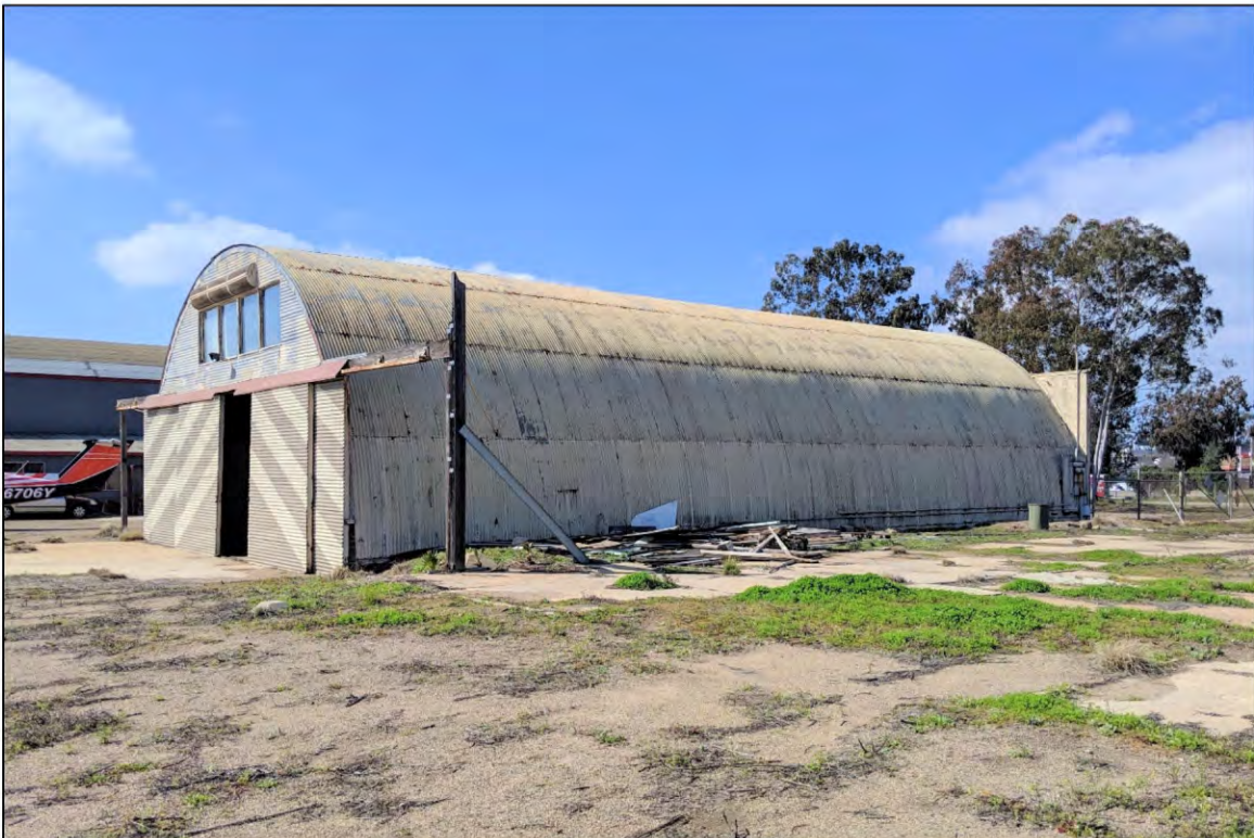
Figure 33: Three-quarter view showing the east and north elevations.
