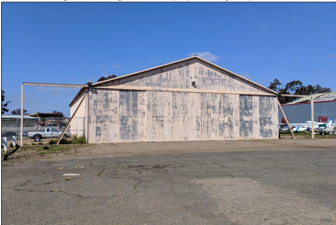
Figure 52: Photo of the east elevation of Building 8.
