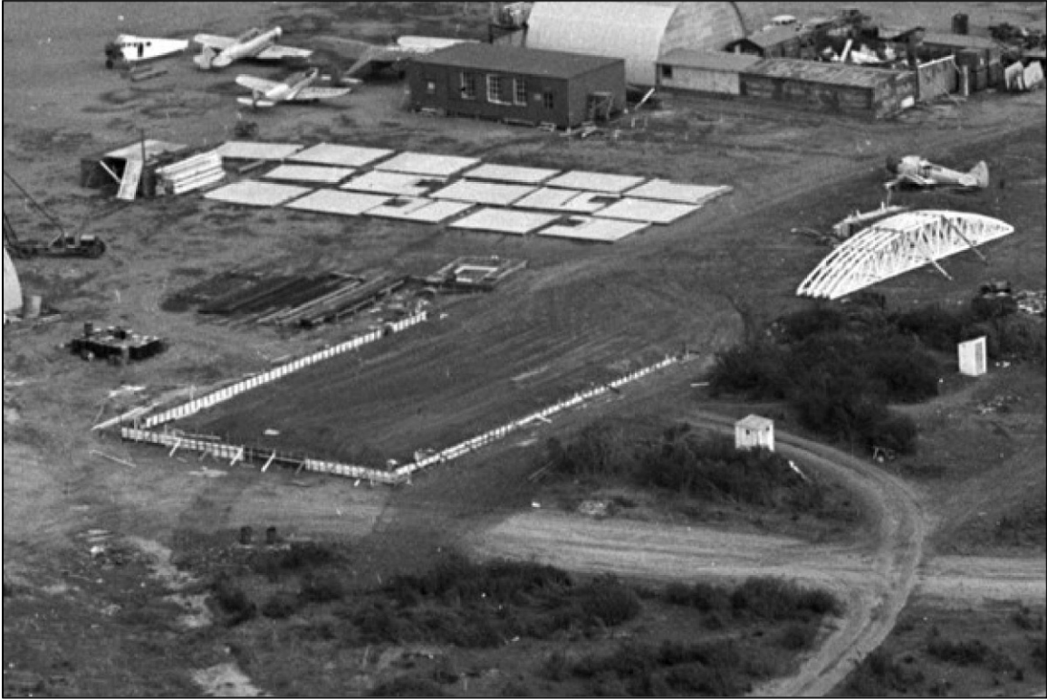
Figure 36: March 1947 photo looking NE. San Diego History Center, UT84_22856.2
