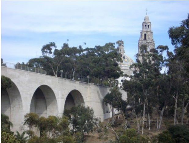
Cabrillo Bridge and Balboa Park
