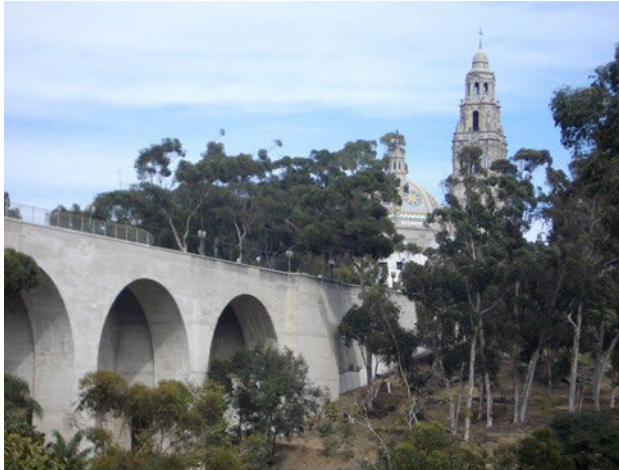
Cabrillo Bridge and Balboa Park
