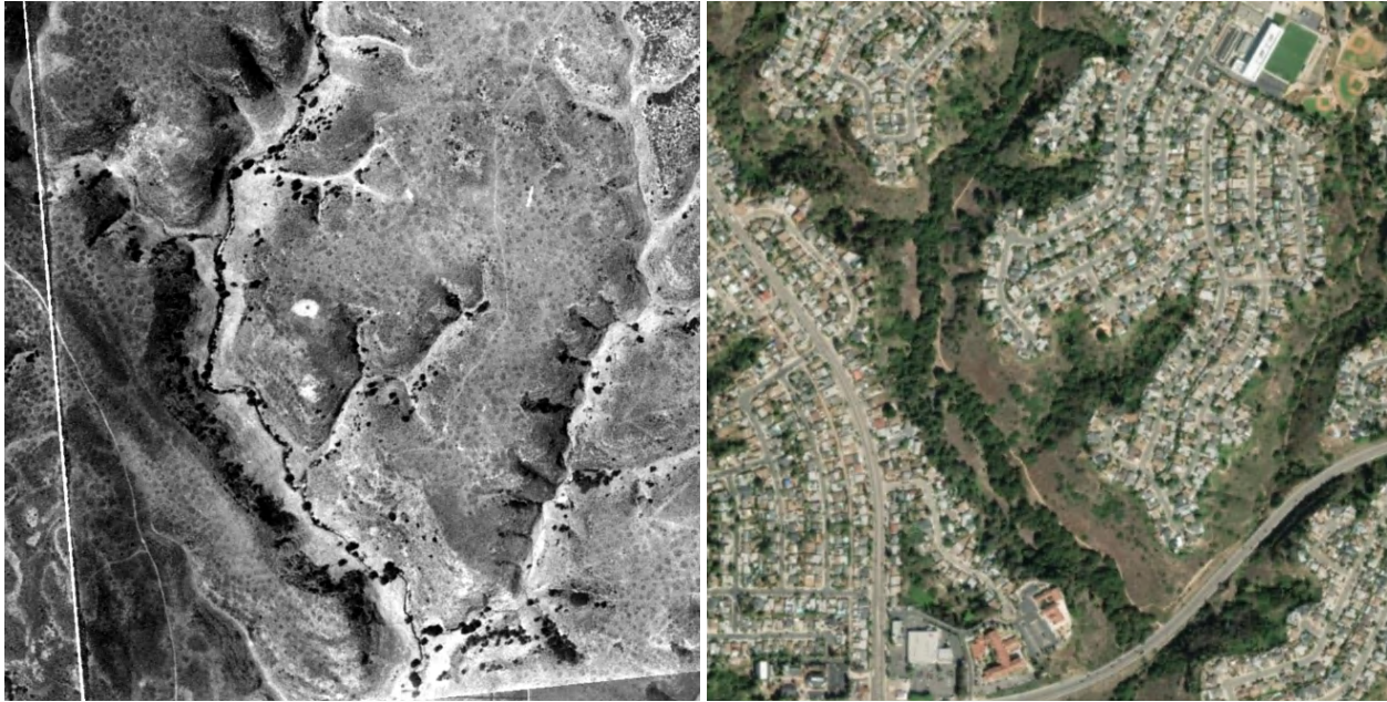
Figure 10. Comparison between the extent of riparian vegetation along Tecolote Creek in historic (left) and modern (right) aerial imagery. Development and urban runoff have caused a shift in streamflow from intermittent to perennial, likely contributing to an increase in riparian forest density ( Left: SDDPW 1928, courtesy of SDDPW; Right: Maxar 2023).
