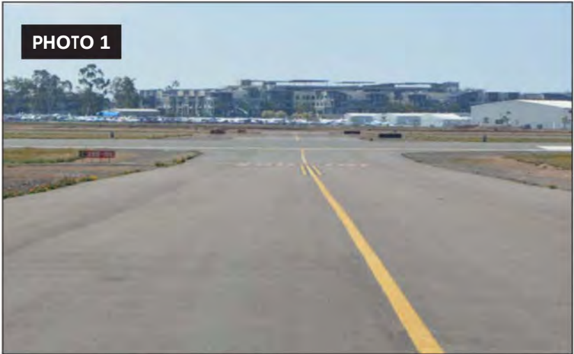
Taxiway C Facing South
