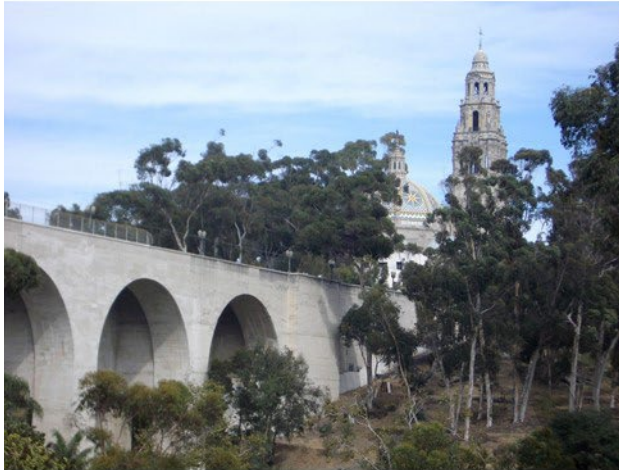
Cabrillo Bridge and Balboa Park
