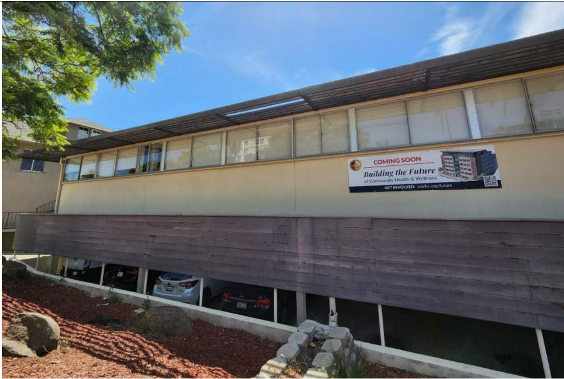
Figure 17: 2660 First Ave, East Elevation from Sidewalk, with structural columns clearly visible below wood fence. (August 2024)
