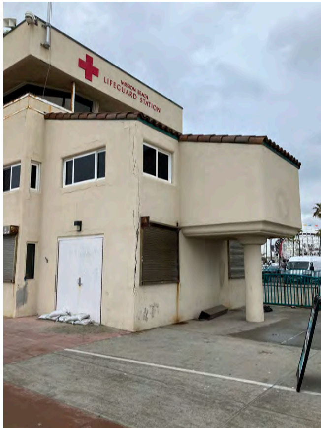
PHOTO 2: SOUTHWEST CORNER OF BUILDING
