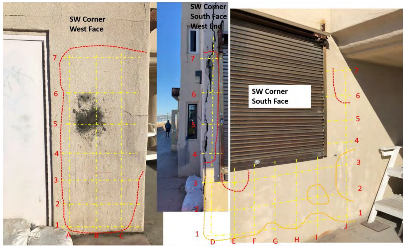
Half-Cell Testing Reference Sketch at Location 2.
