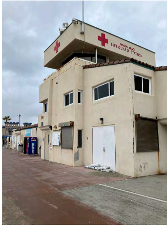
PHOTO 1: WEST FACE OF BUILDING
