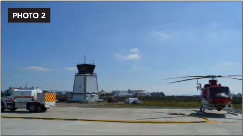
Air Traffic Control Tower
