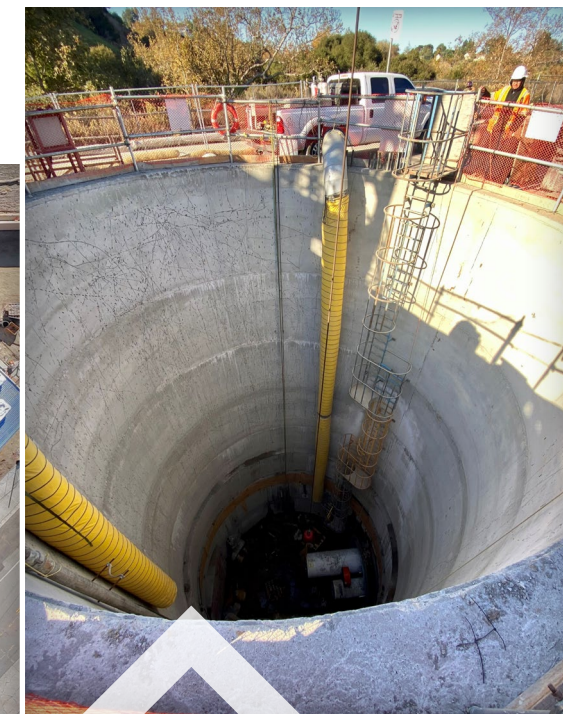
Morena Conveyance Northern Pipelines and Tunnels Project
