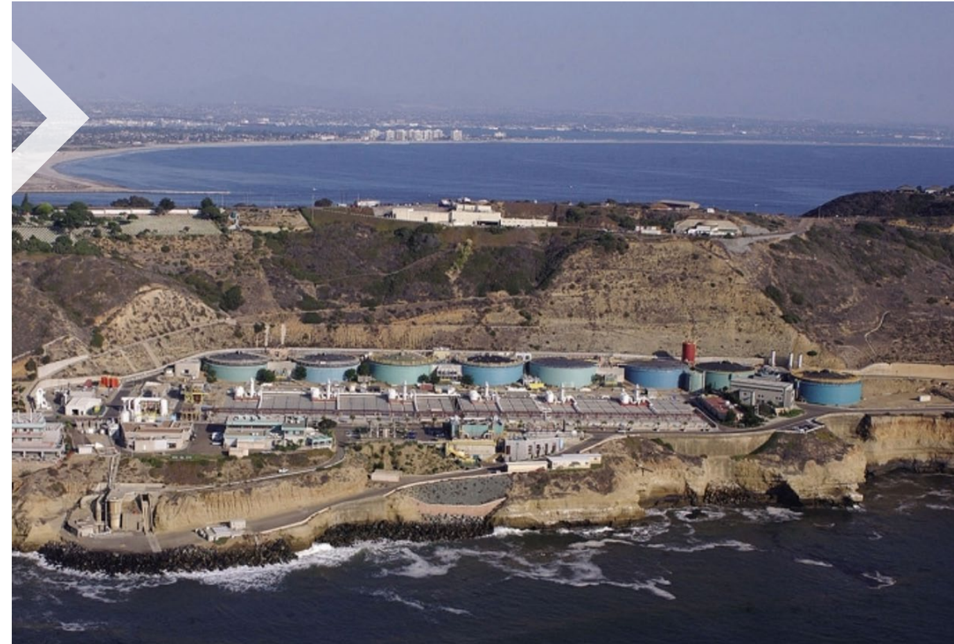
Point Loma Wastewater Treatment Plant
