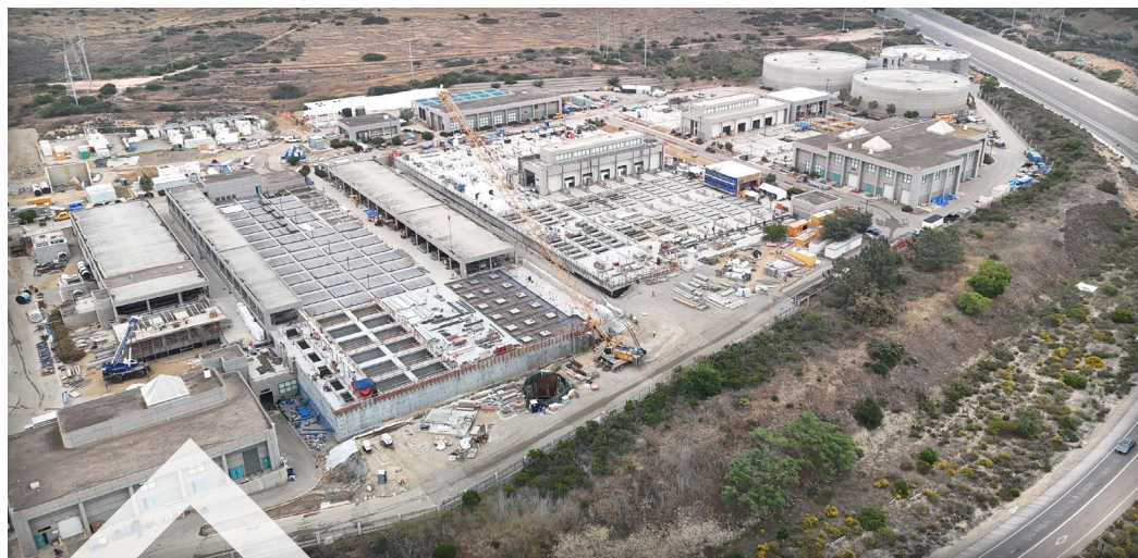
North City Water Reclamation Plant Expansion
