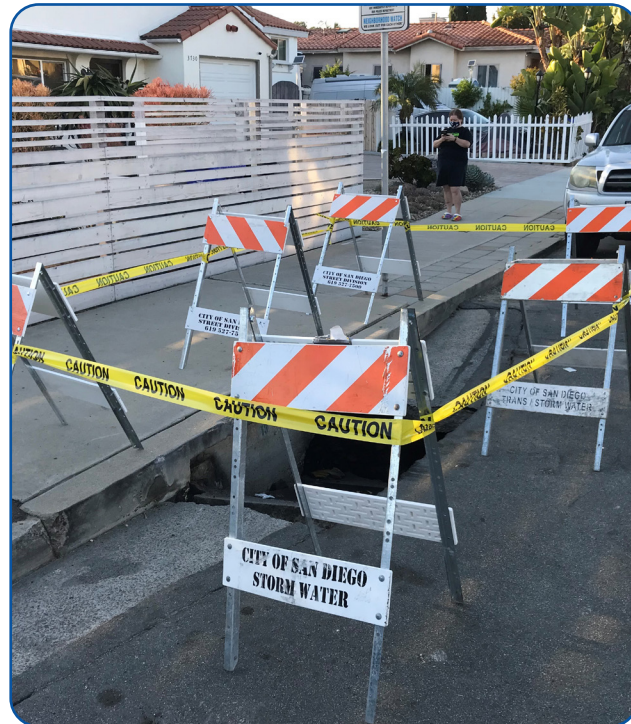
Blocked off sinkhole at 3730 Mississippi St in the Pueblo Hydraulic Unit due to storm drain infrastructure deficiency.
