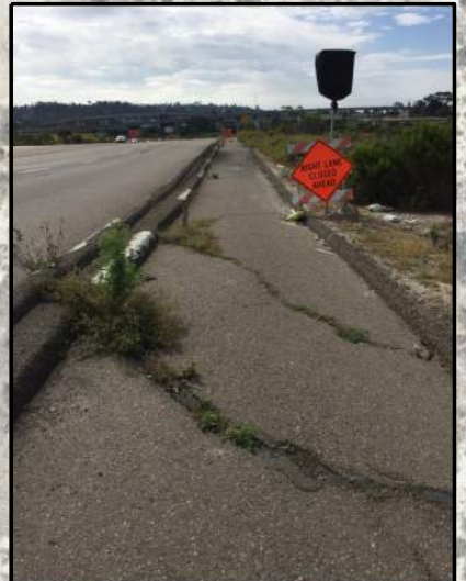
2 FRIARS ROAD CYCLE TRACK PAVEMENT IN POOR CONDITION (LOOKING SOUTH)
