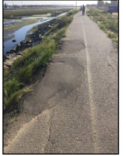
2 PAVEMENT FOR SHARED-USE PATH IS IN POOR CONDITION (LOOKING EAST)
