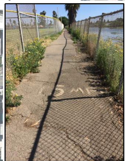
1 2 3 EXISTING PAVEMENT IN POOR CONDITION AND SHARED BIKE PATH IS NARROW IN WIDTH (LOOKING SOUTH)
