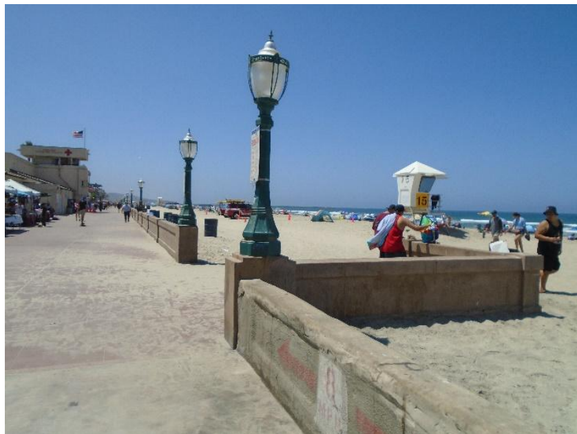
Figure 2: In 2016, stairs were removed and beach access was modified with L-shaped openings in the seawall. Photo from section originally completed in 1925, appears in blue on Figure 1. (July 2021, DSC03046).
