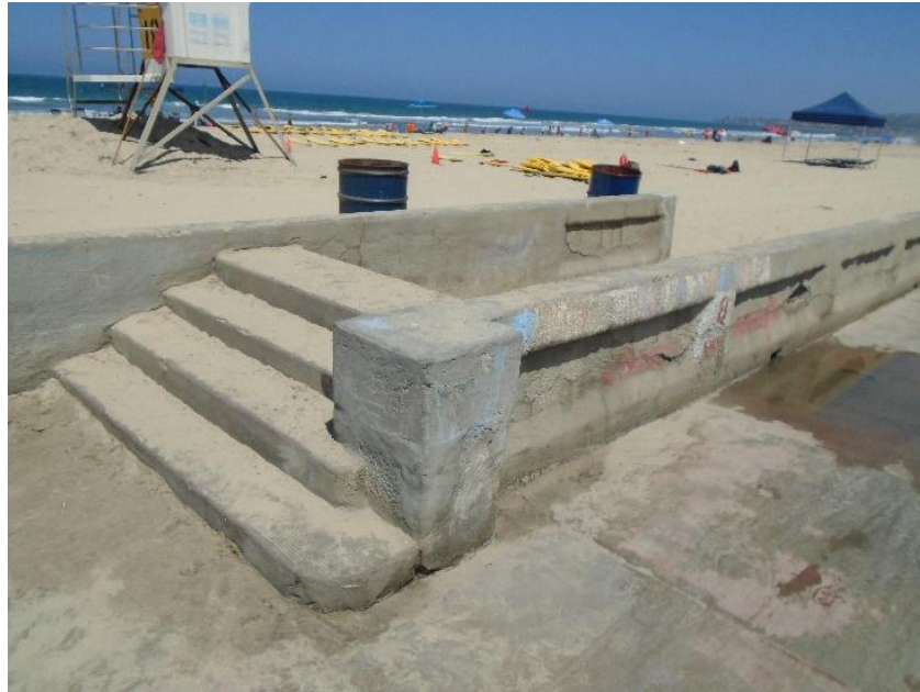
Figure 1: Integrated stairs originally provided access to the beach. Photo from section completed in 1928, appears in yellow on Figure 1. (July 2021, DSC03046).
