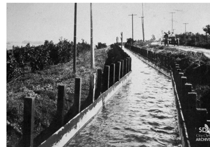
Flume to transport water to San Diego from Cuyamaca Mountains, 1905, City of San Diego City Clerk's Archive
