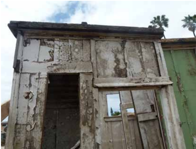
P14 - West Elevation (5 / W1), door 102 (1'-10" x 6'-2"), no door, part of the non-historic addition)
