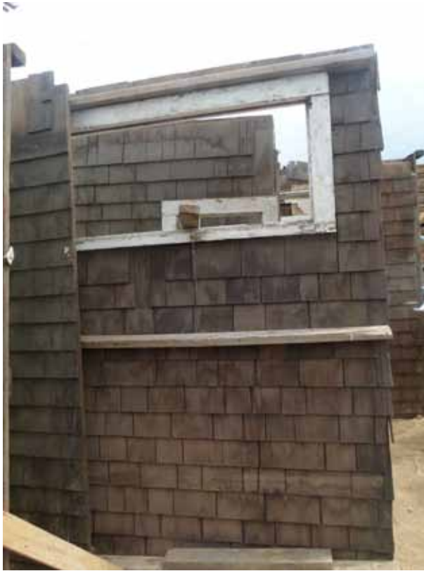
P24 - East Elevation (28 / E3-2), window missing
