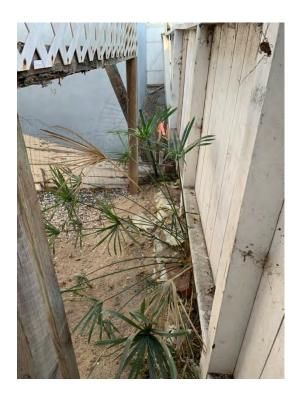
**South** Corner of Lot 5 photo, here you can see that there is <u>also</u> no slope or grade of any kind, and that the Lot 19 retaining wall is 2.5 feet above the existing Lot 5 grade of about 33.4', or at about 36.28' elevation according to Lot 19 survey.
