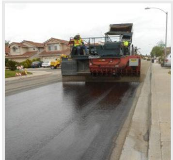
Slurry seal is applied after the crushed rock layer has cured for 3 days
