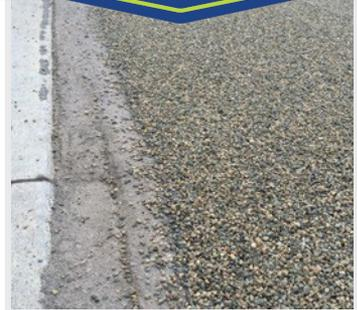
Completion of crushed rock layer prior to slurry seal application
