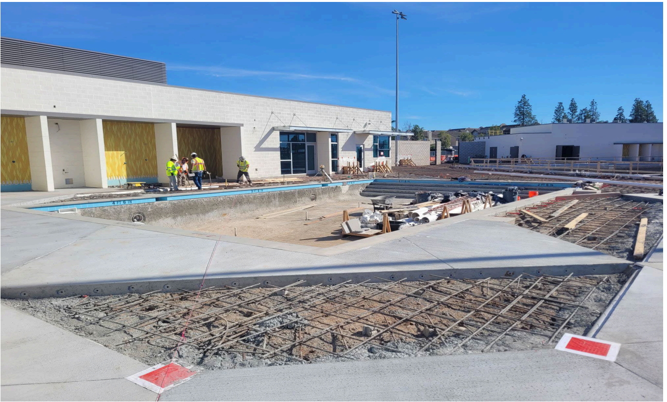
Concrete placement for pool deck area
