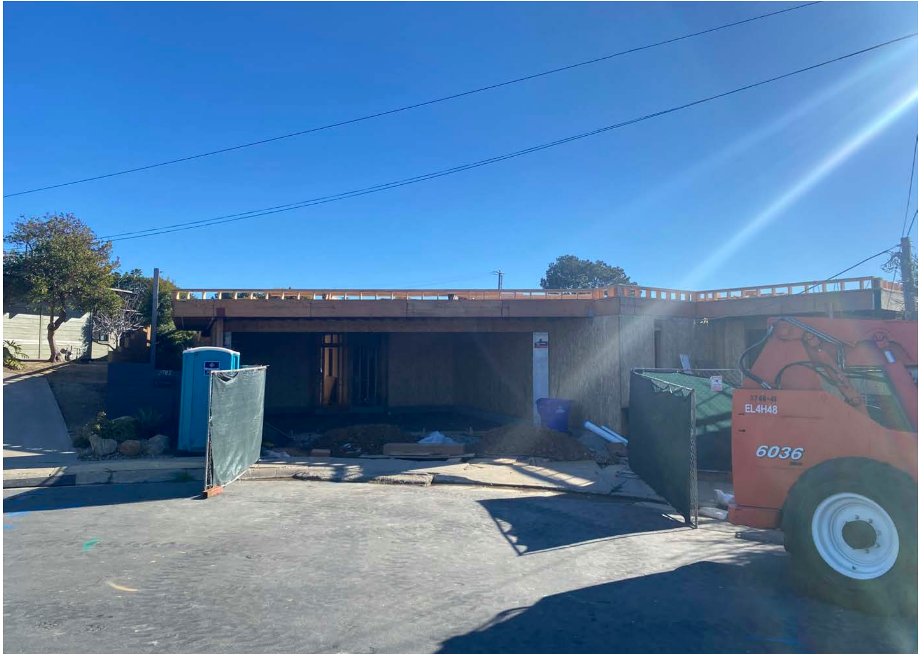
10 - 2702 BORDEUAX AVE, LA JOLLA, CA 92037- UNDER CONSTRUCTION
