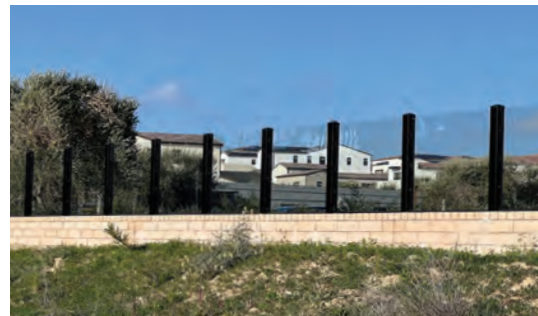
Example Photo of Solid View Wall / Fire Rated Wall With Fire Rated Glass Block
