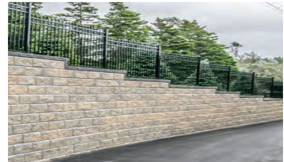
Example Photo of Iron Fence Theme Wall
