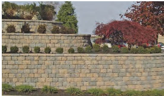
Example Photo of Masonry Theme Wall
