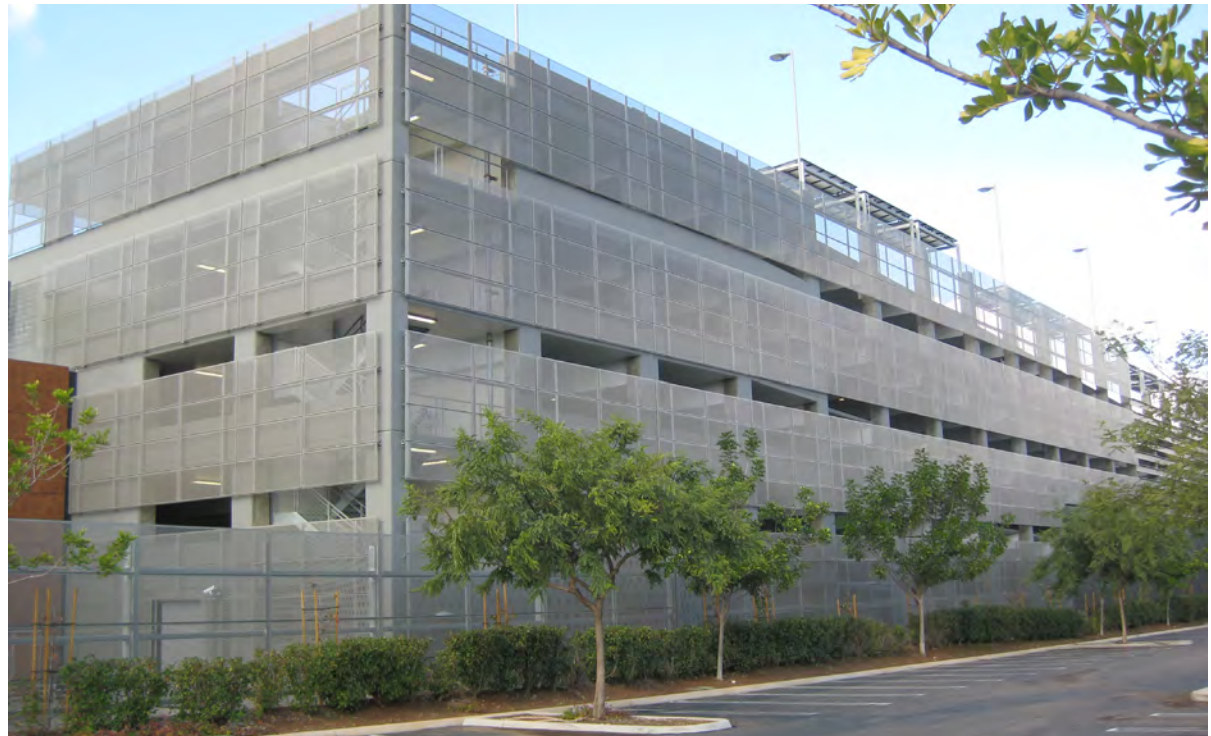
A typical parking garage
