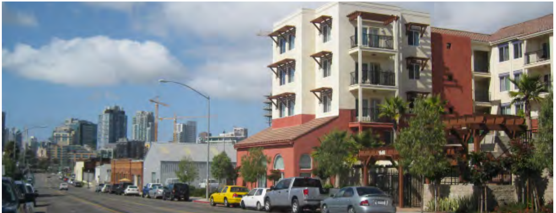
National Avenue view corridor
