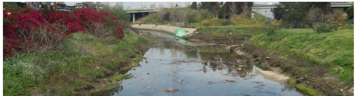
Las Chollas Creek in need of restoration
