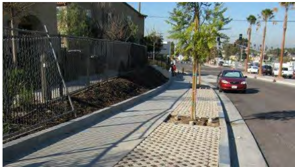
Provide storm water infiltration in parkways
