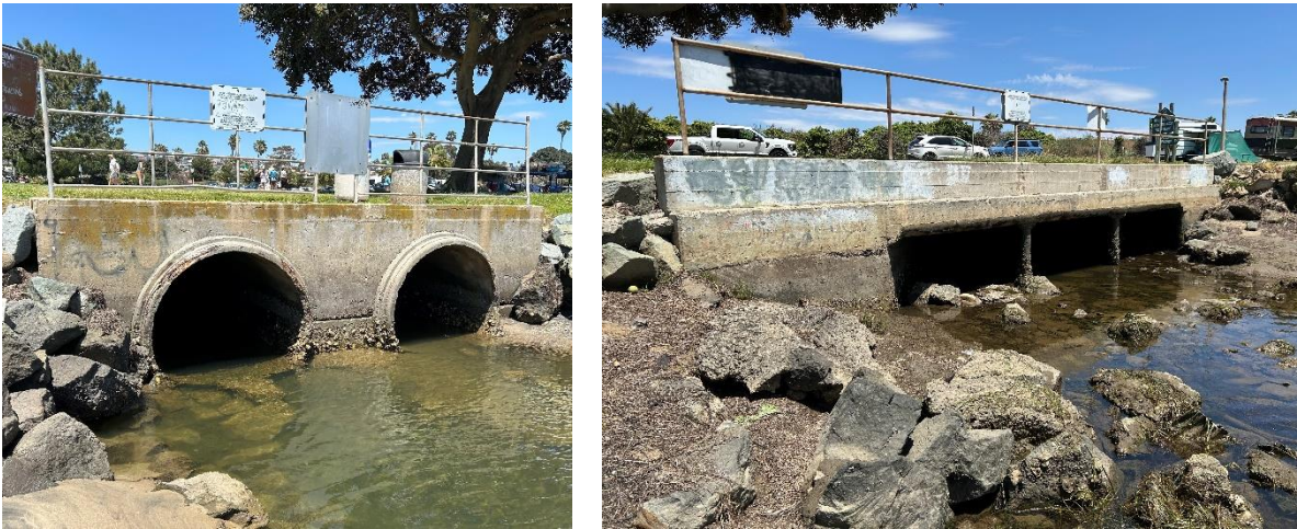
Figure 2-1. Existing Storm Drain Outfalls
