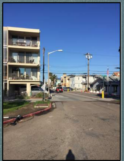
2 NO PEDESTRIAN FACILITY ON THE NORTH SIDE OF SANTA CLARA PLACE THEREFORE CYCLISTS AND PEDESTRIANS MUST USE ROADWAY (LOOKING WEST)
