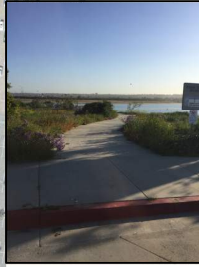
1 SHARED USE PATH BEGINS, MISSING ADA CURB/BIKE RAMP TO ENTER FACILITY (LOOKING NORTH)
