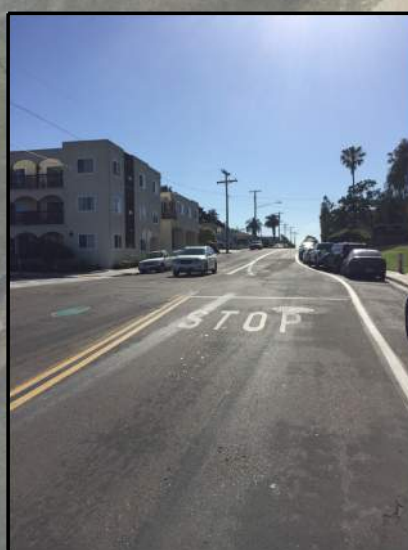
1 MISSING WAYFINDING SIGNAGE FOR CYCLISTS TRAVELING WESTBOUND ON PACIFIC BEACH DRIVE (LOOKING WEST)
