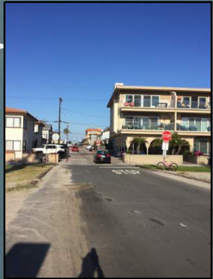
1 MISSING CONNECTIVITY FOR PEDESTRIANS TO TRAVEL FROM BAYSIDE WALK TO EL CARMEL POINT (LOOKING WEST)
