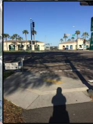
1 SHARED PATH ENDS WITH INADEQUATE WAYFINDING SIGNAGE (LOOKING WEST)
