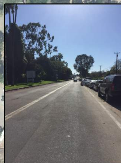
2 3 MISSING CONNECTIVITY, NO SIDEWALK ON SOUTH SIDE OF PACIFIC BEACH DRIVE AND PEDESTRIAN/CYCLISTS MUST USE ROADWAY (LOOKING WEST)
