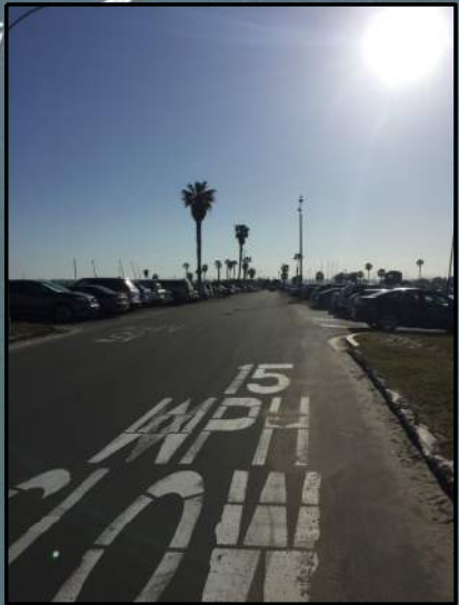
2 LACK OF PEDESTRIAN FACILITIES SUCH AS A SIDEWALK PRESENTS A SAFETY CONCERN (LOOKING EAST)
