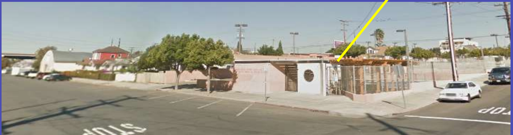
Barrio Station Outdoor Swimming Pool (City of San Diego Property)
