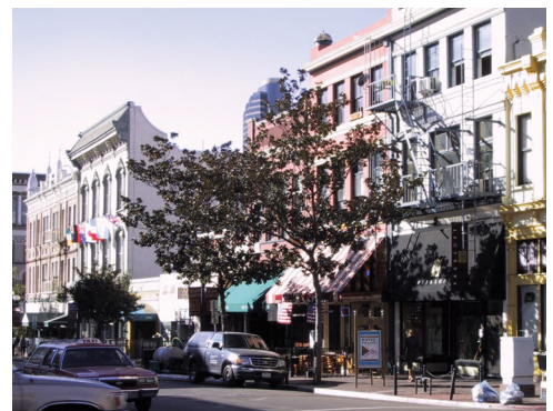
Horizontal (top) and vertical (middle) articulation is important to lend a human scale to larger developments. The small parcels of the Gaslamp Quarter (above) produce visual variety at street level.
