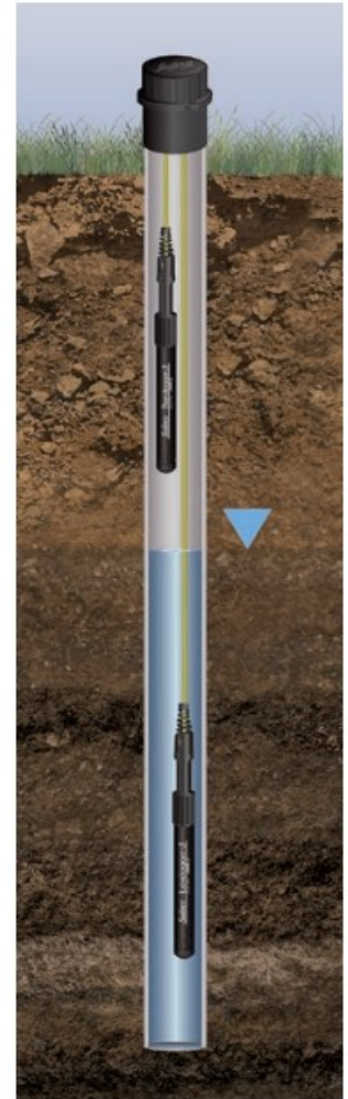
Barologger 5 and Levellogger 5 installed in Well Using L5 Direct Read Cables
