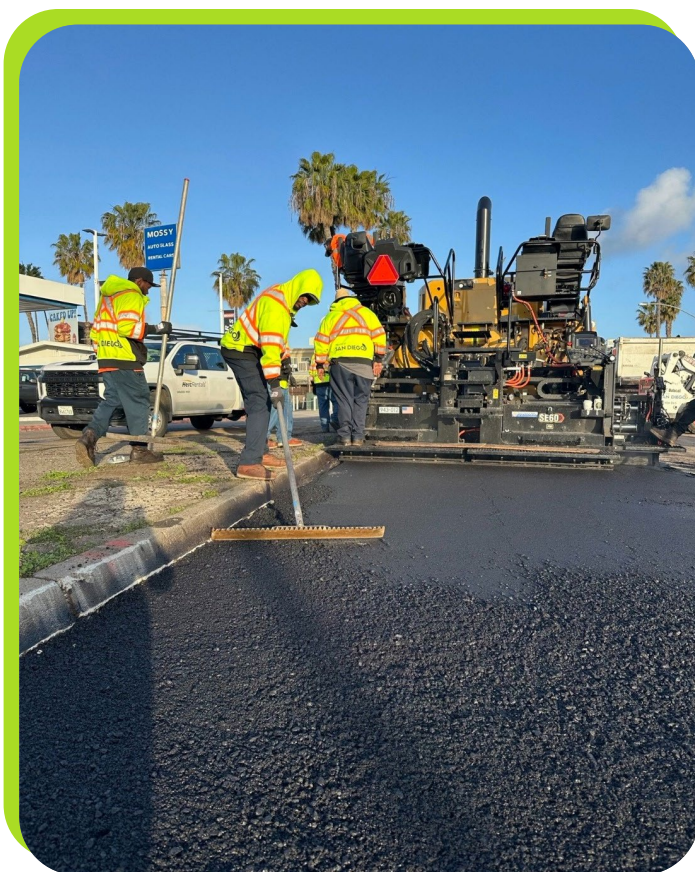
City crews completing asphalt finishing work as part of in-house rehabilitation efforts.
