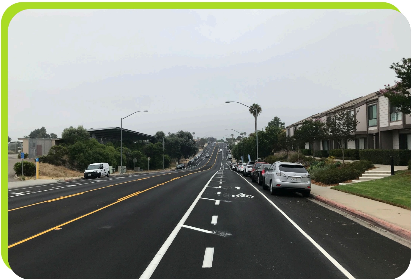
Street resurfacing and striping improvements enhancing pavement condition and roadway safety
