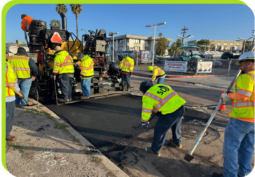
In-house paving crew conducting curb-to-curb rehabilitation, improving localized street conditions.
