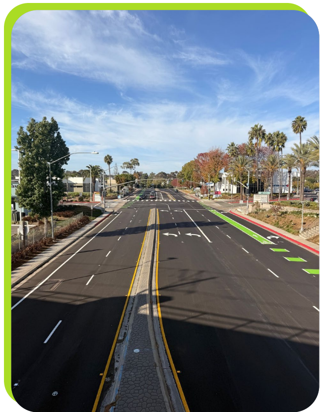
Completed roadway resurfacing project enhancing ride quality, safety, and multimodal striping.
