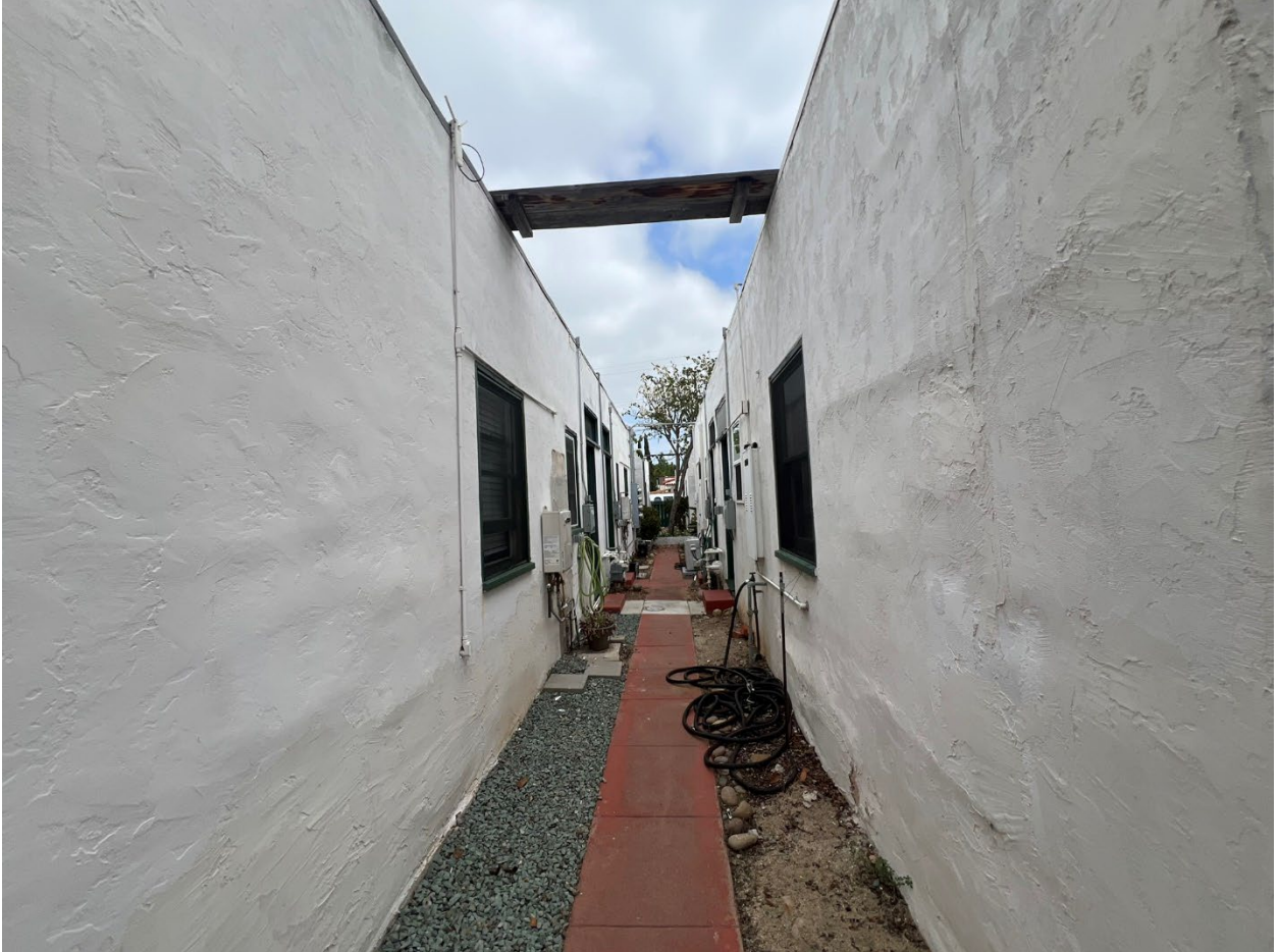
Overview of walkways between semi-detached bungalow courts showing east and west elevations (camera facing north)
