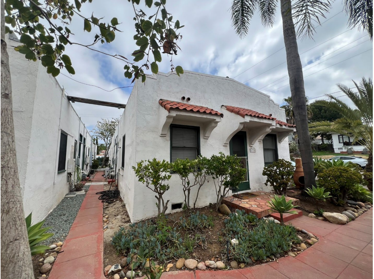
Overview of south and east and west elevations of semi-detached bungalows (camera facing northeast)
