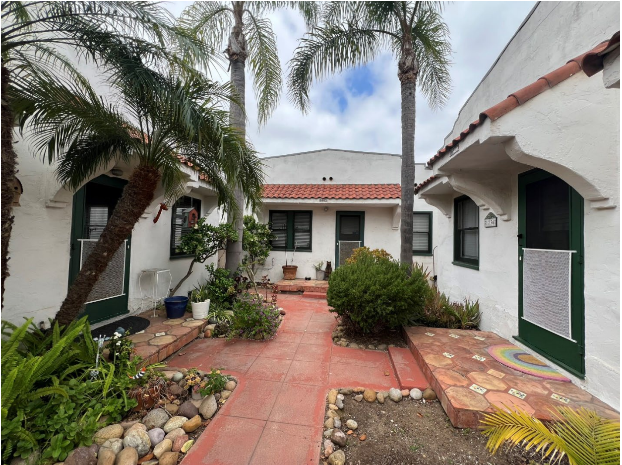
Overview of east elevation of detached bungalow, and the south elevation of the semi-detached bungalow (right) and the north elevation of the detached bungalow (left) (camera facing west).
