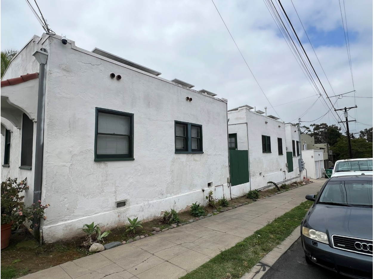
Overview of north elevation of detached bungalows, fronting Elm Street (camera facing southwest)
