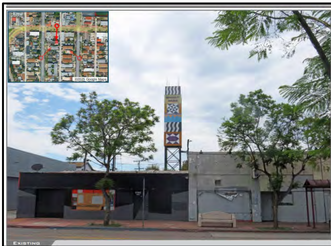
Figure 1 Existing community tower view from 35 th St
