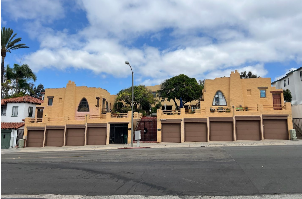
Overview of south elevation and garage area fronting Adams Avenue (camera facing north)
