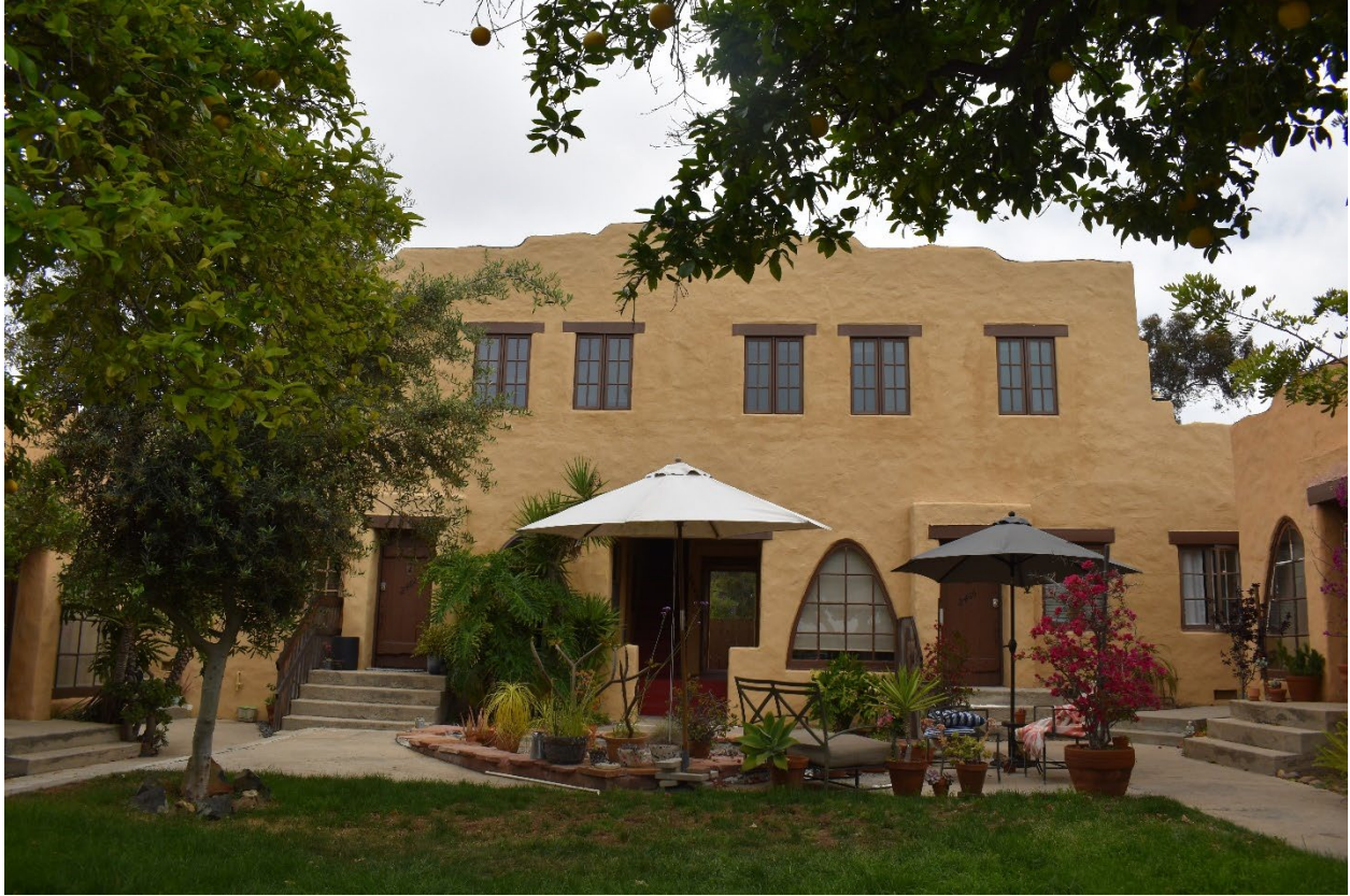
Overview of south elevation of two-story attached bungalow (camera facing north)
