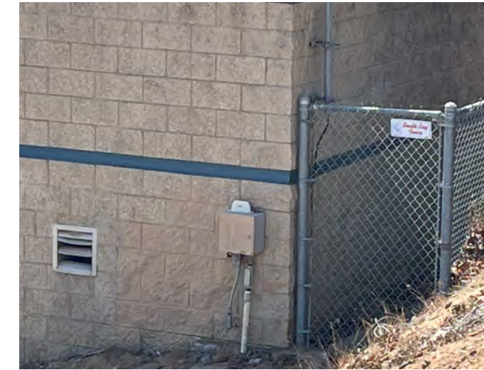
View of northwest corner of existing utility building.
