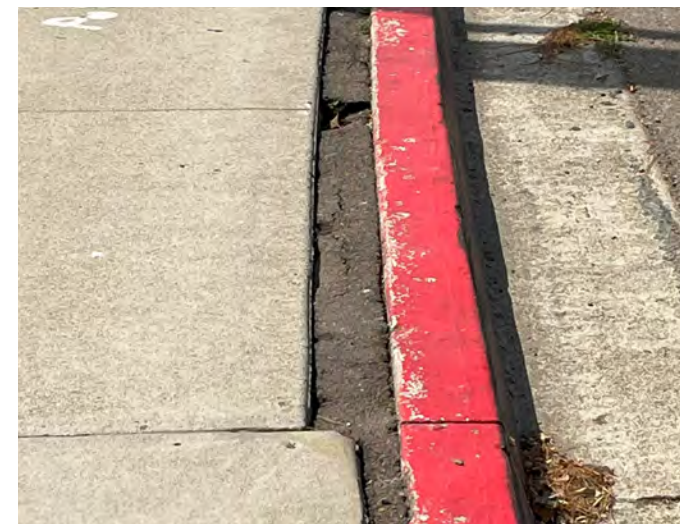
Existing concrete curb.
