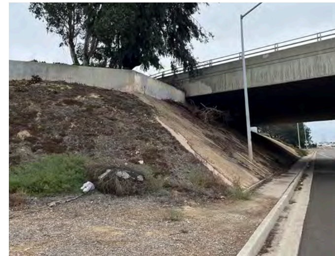
Existing bridge abutment .
