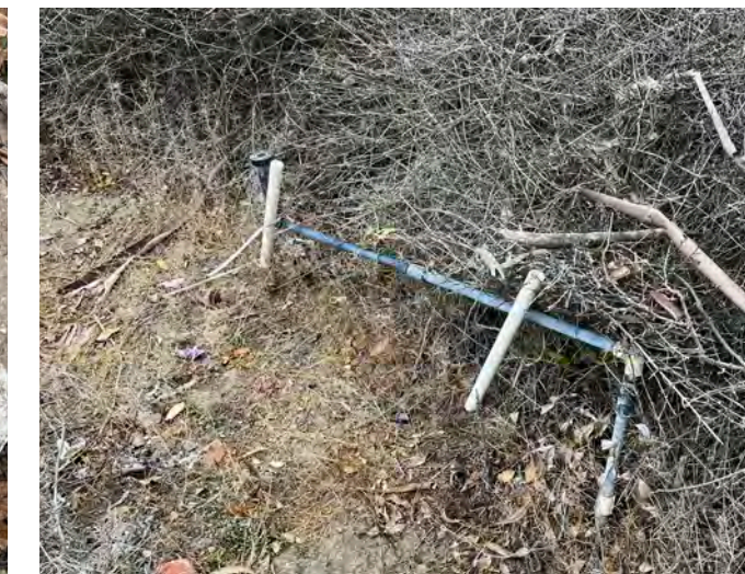
Existing irrigation piping and spray heads within landscape area.
