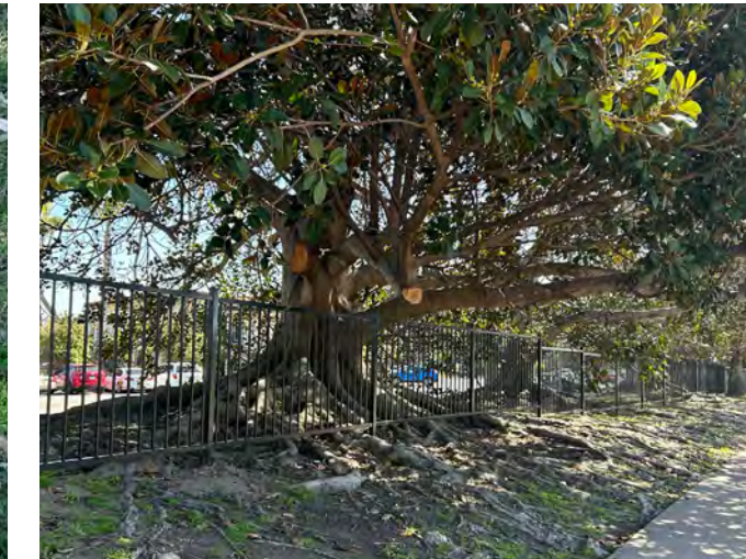
Existing ficus trees adjacent to Bahia Resort. Tree roots have overtaken landscape area.
