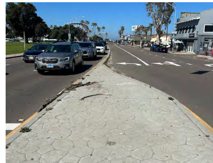
Existing median within this scope area consists of stamped concrete paving.
