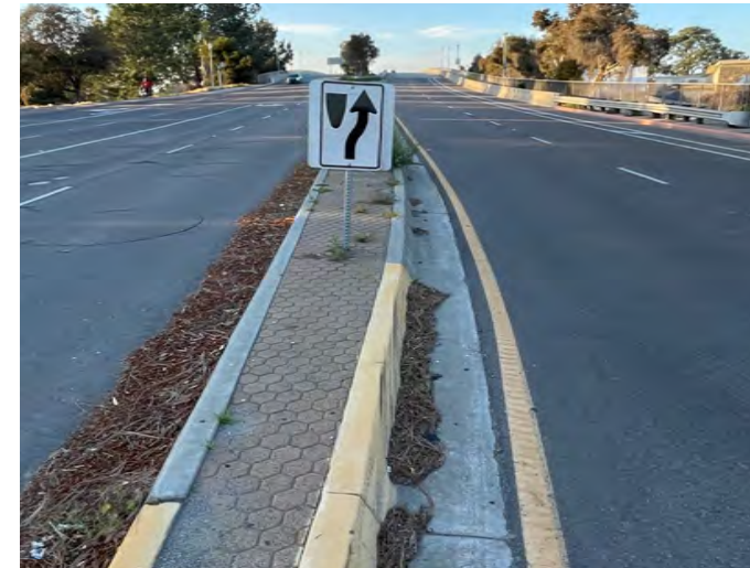
Existing stamped concrete within median.
