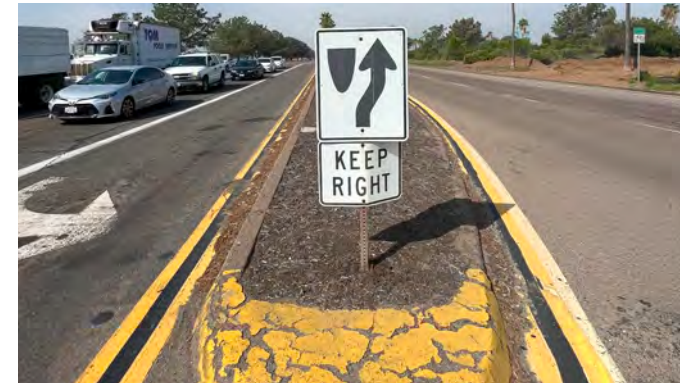
View of median facing west along Sea World Drive.
