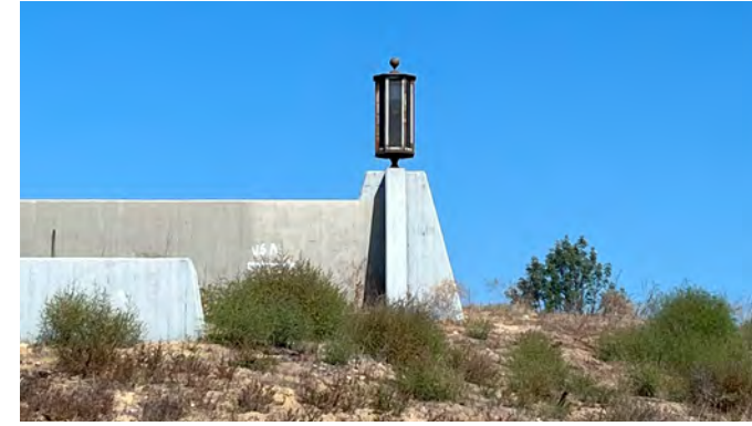
View of historic lantern on Sunset Cliffs Bridge.
