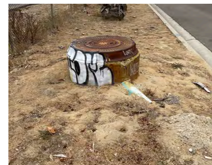
Existing sewer line running along east side of Mission Bay Drive under existing palm trees.
