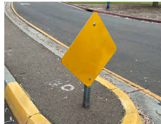
Existing medians within this scope area consist of AC paving.
