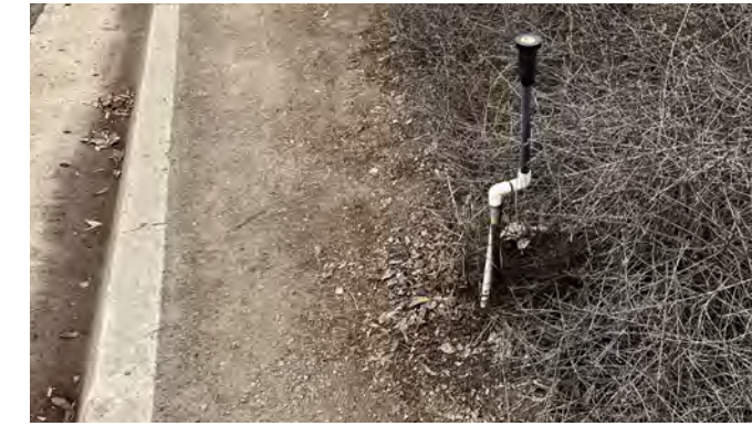
Existing irrigation and degraded landscape area facing north towards Mission Bay Drive.
