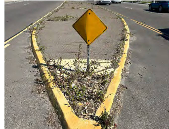
Existing medians with AC paving.
