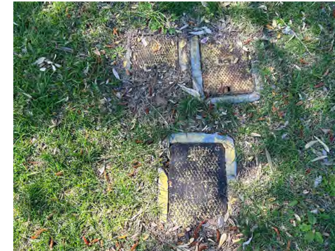
Existing irrigation valve boxes.
