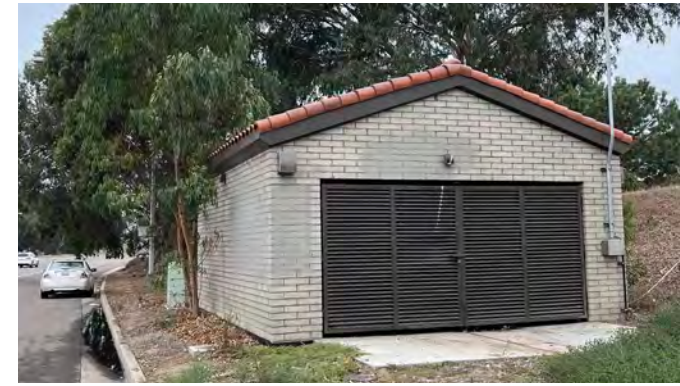
View from Mission Bay Drive facing northwest towards utility building.
