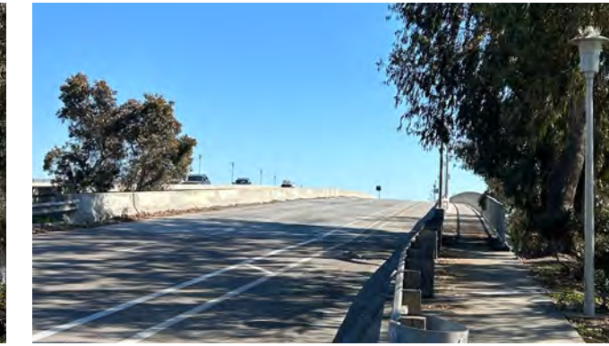
View from north of the bridge facing south towards the median.
