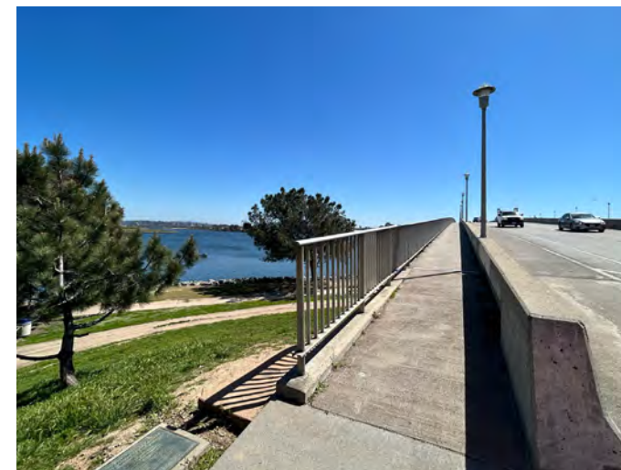
Existing pedestrian walkway along Ingraham Street Bridge.
