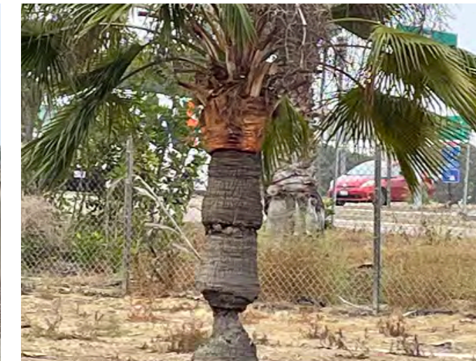
Existing palm tree condition in landscape areas along Mission Bay Drive.
