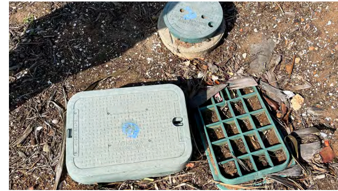
Existing irrigation valve boxes in median.
