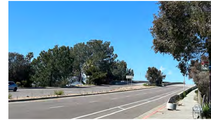
View from south of the bridge facing northwest towards center median.
