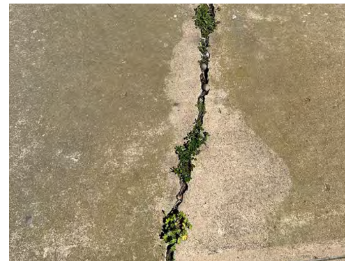
Existing concrete paving.
