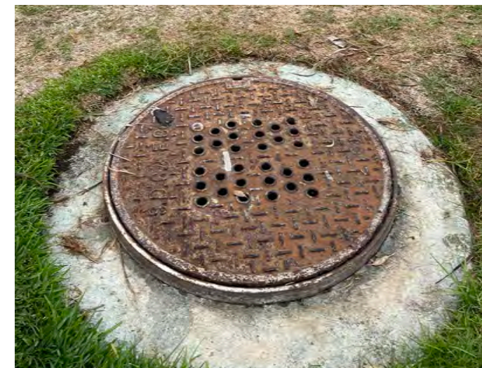
Existing manhole and utilities on west side of Mission Bay Drive
