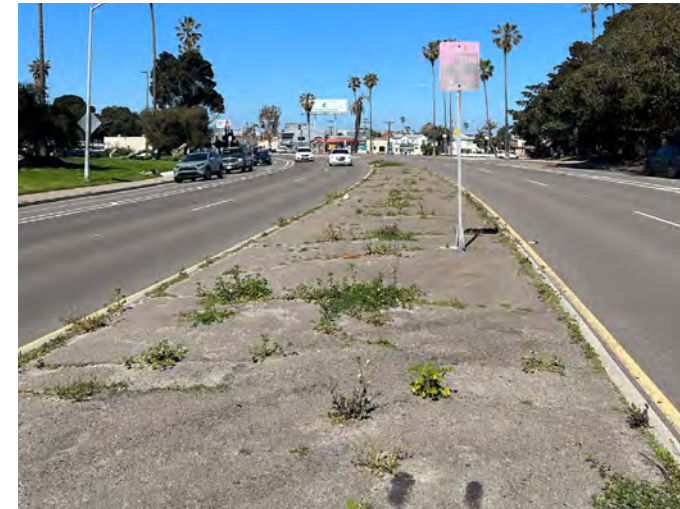
Existing medians within this scope area consist of AC paving.
