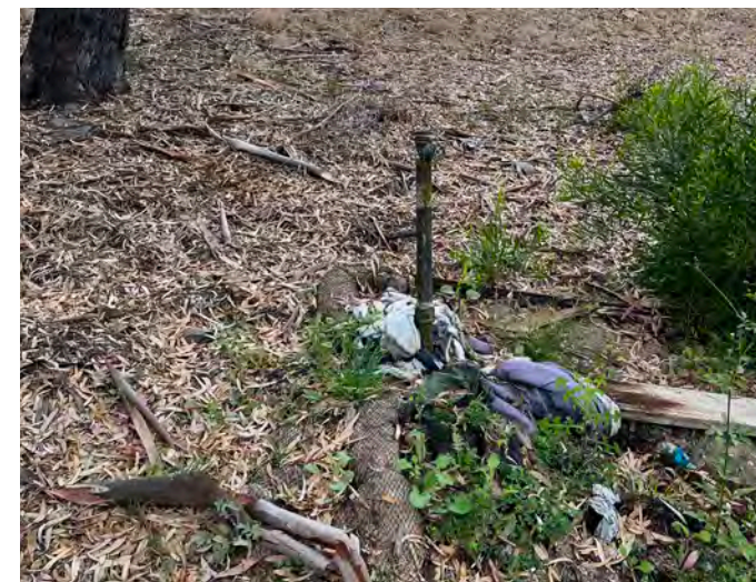
Existing irrigation and debris in landscape area.
