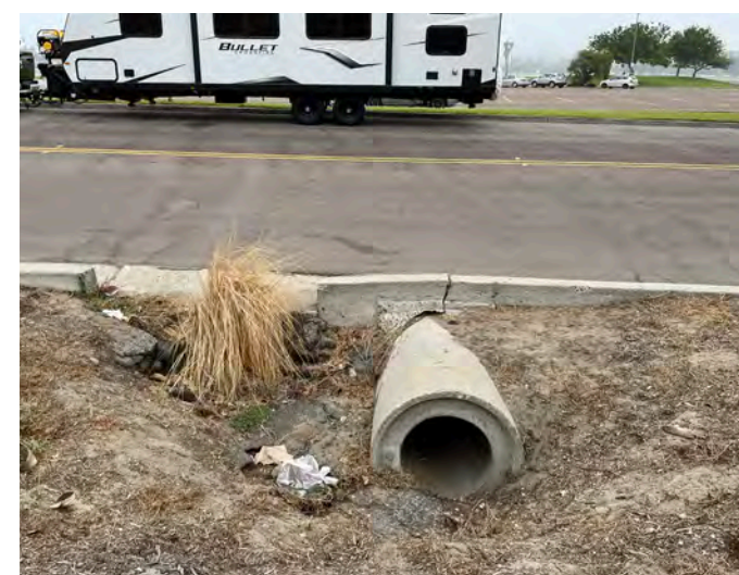
Existing drainage culvert at Mission Bay Drive.
