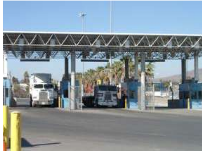
Truck Inspection at Otay Mesa POE
