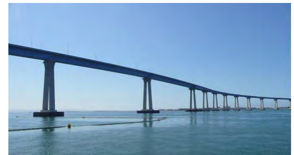
The San Diego Coronado Bay Bridge built in the 1960s
