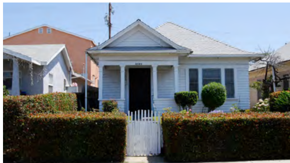
Enclosed front yards of historic homes along Newton Avenue
