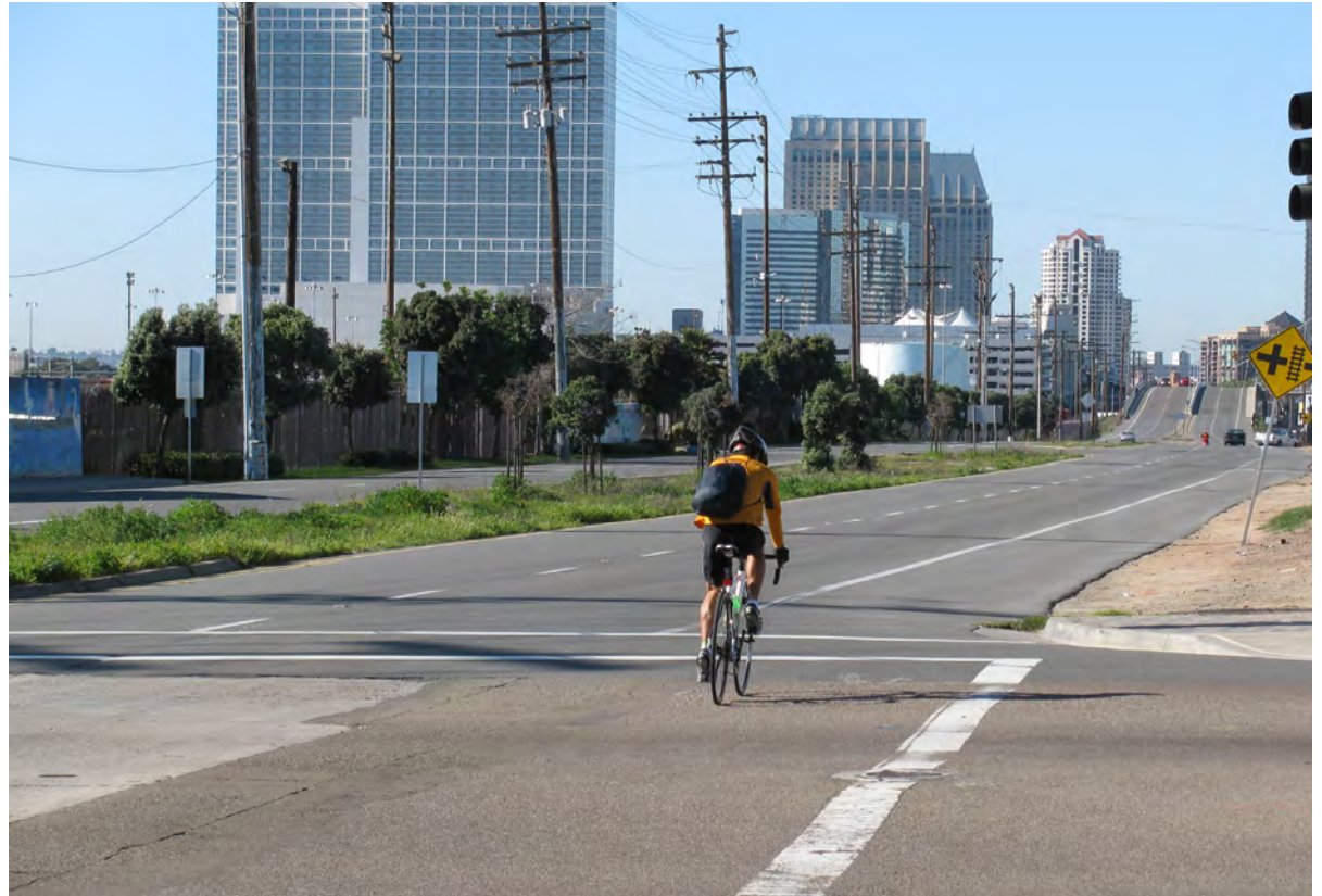
Bike lane along Harbor Drive
