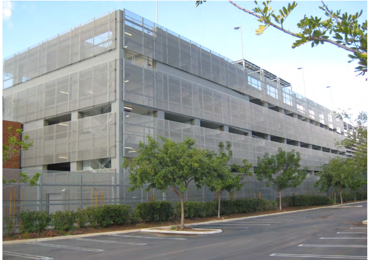
A typical parking garage
