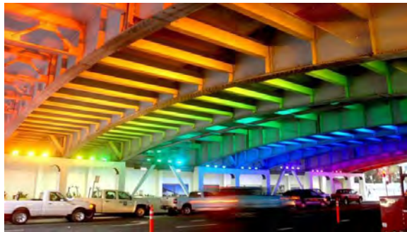
Retrofitting freeways with architectural lighting
