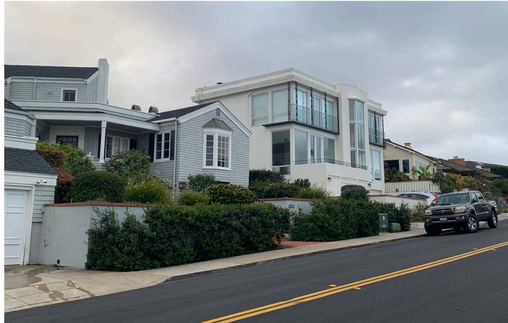
EXISTING BUILDING - VIEW FROM DOWNHILL SIDE OF SPINDRIFT DRIVE
