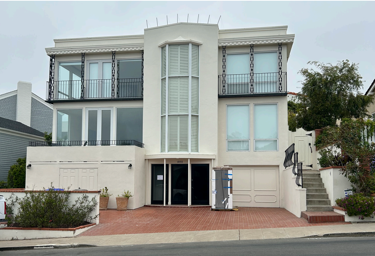
EXISTING BUILDING - FRONTAL VIEW FROM PUBLIC RIGHT OF WAY
