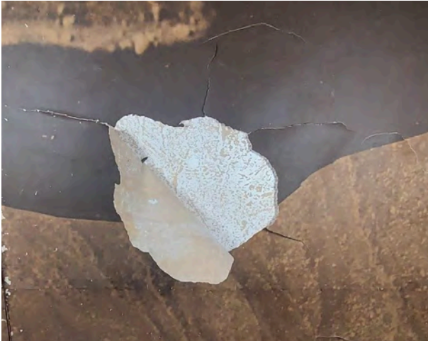
Figure 39: West Wall - Before Treatment (Detail).
