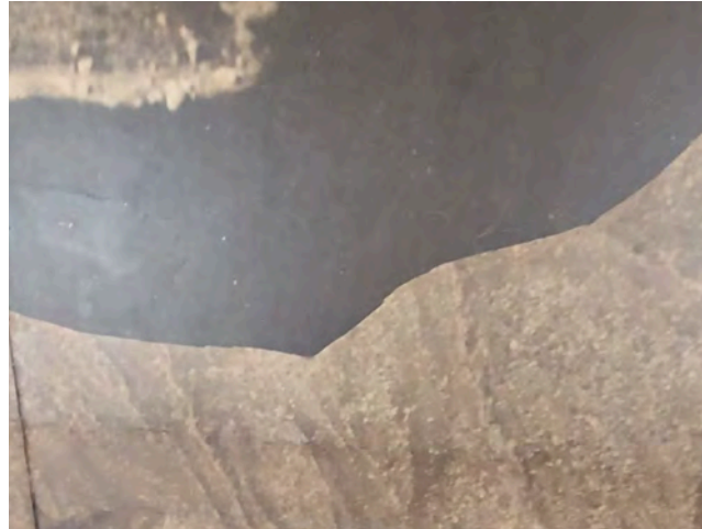
Figure 40: West Wall - After Treatment (Same Area Detail).
