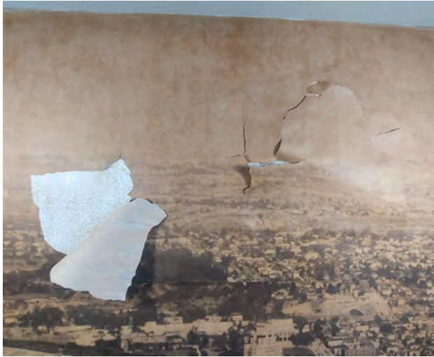
Figure 43: West Wall - Before Treatment (Detail).
