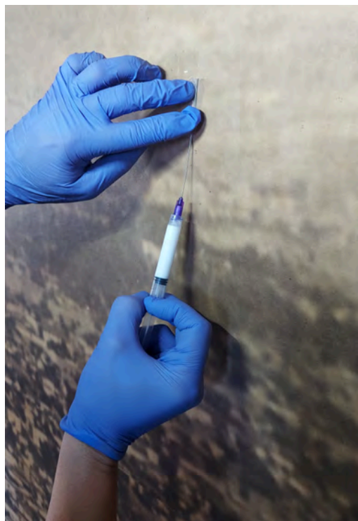
Figure 28: Adhesive was applied using narrow syringes when access was limited.
