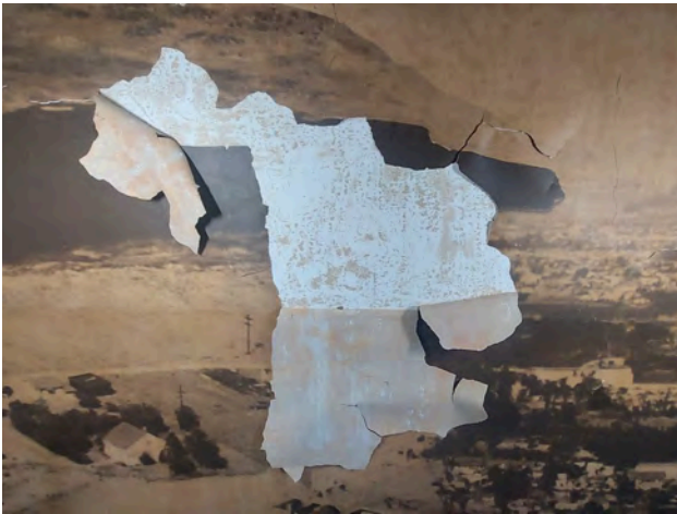
Figure 41: West Wall - Before Treatment (Detail).
