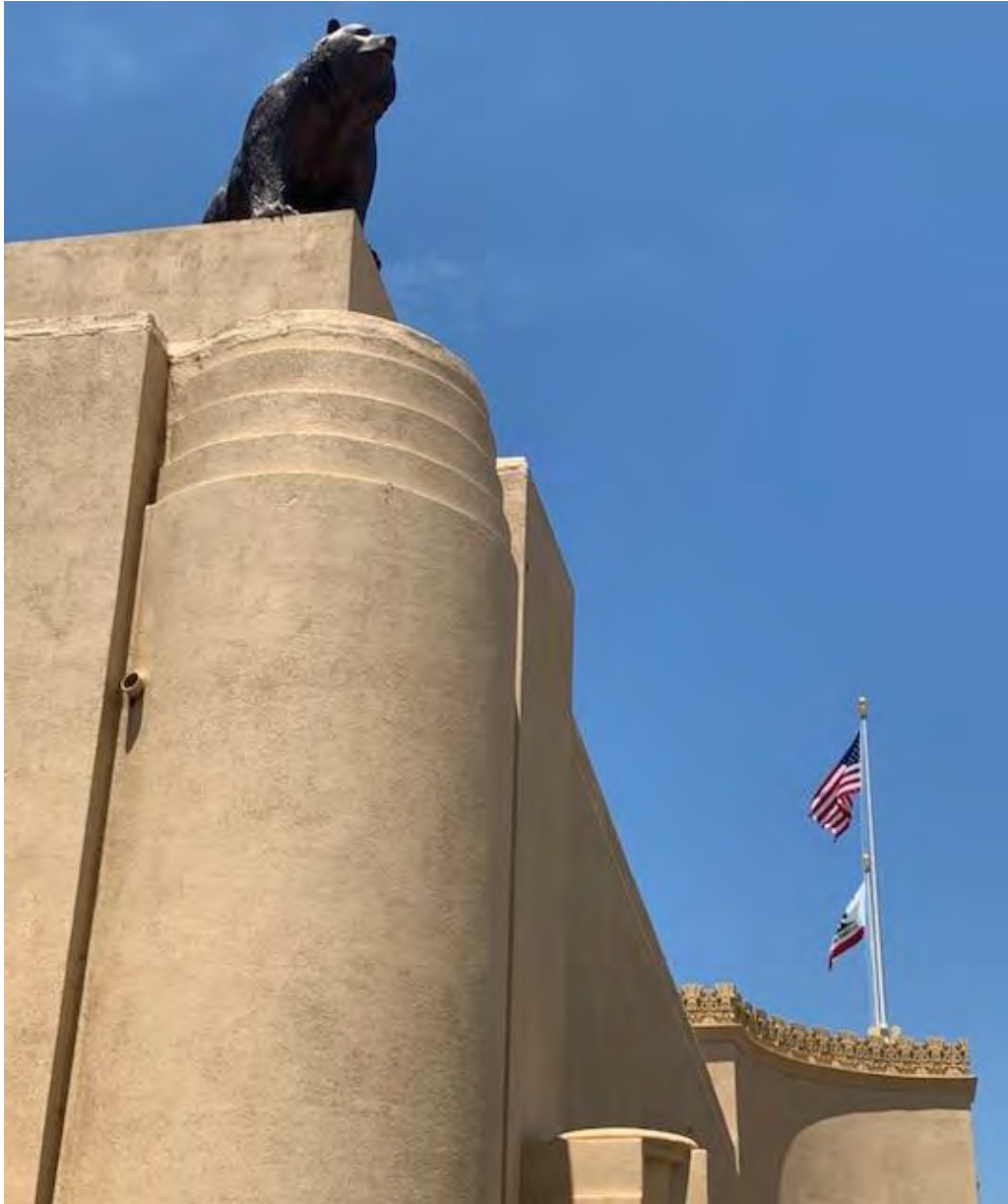
Installed reconstructed California grizzly bear sculpture at roofline corner of the California State Building. The bear's forepaws extend over the curved parapet edge, replicating the original 1935 silhouette and reinforcing the building's vertical sculptural emphasis. Flagpoles are visible in their restored historic locations.
