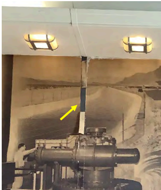
Figure 19: Corrosion of the metal joint led to detached sections of the paper (East Wall)
