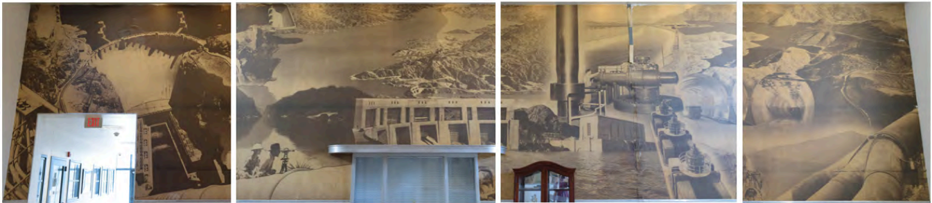
East Wall – Before Treatment
