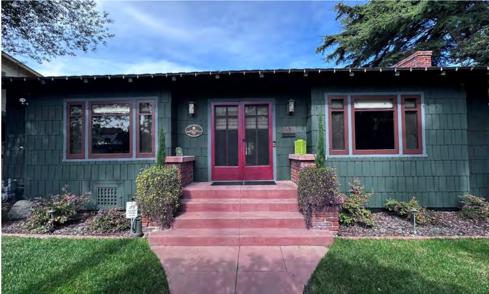
Photo of current home: Front Elevation
