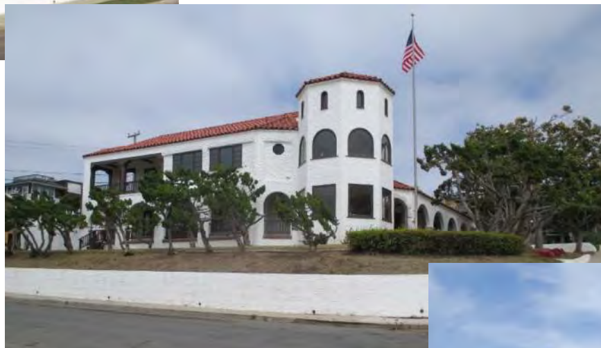
Before: Existing home prior to construction
