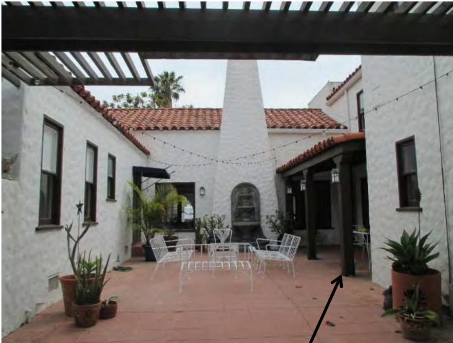
Before Non-original tiled patio cover
