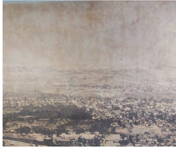
Figure 44: West Wall - After Treatment (Same Area).
