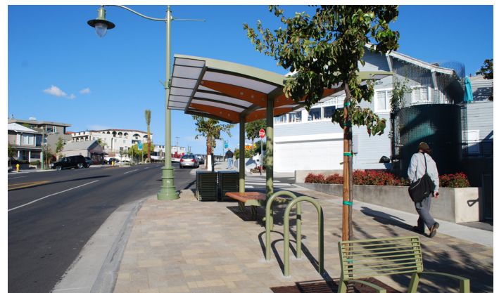
An Enhanced Bus Stop Includes Curb Extensions, Shelter, Bicycle Racks, Seating, Lighting, and Landscaping
