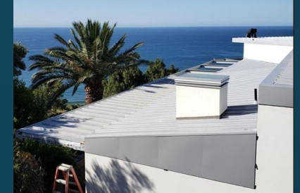
Standing Seam Metal Roofing
