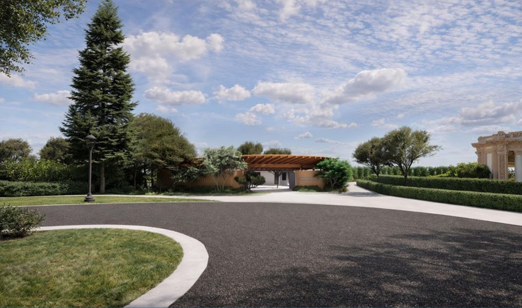
View from north of public restrooms
