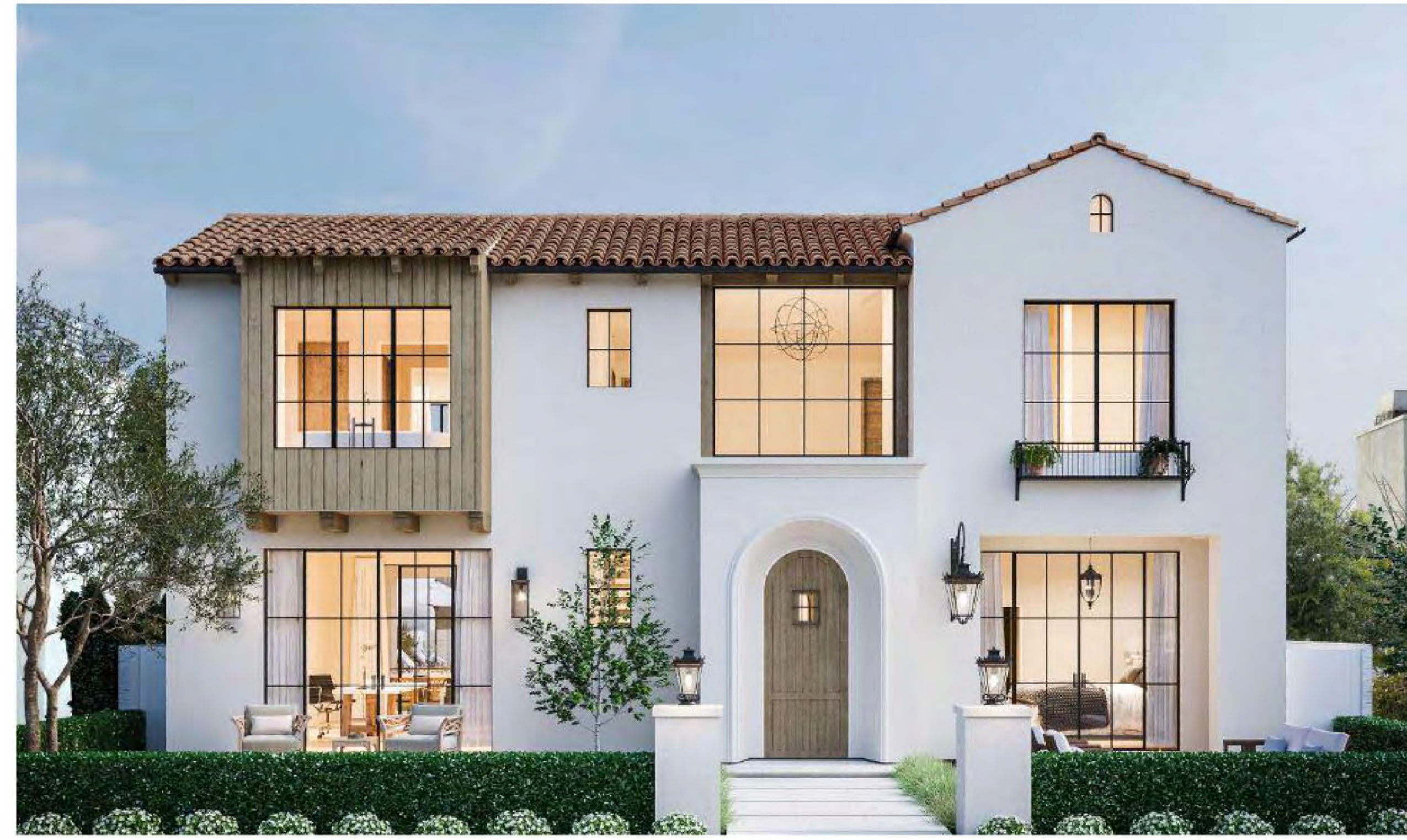
ENTRY DOOR/STUCCO ARCH DETAIL, METAL WDW, WOOD SIDING INSPIRATION
