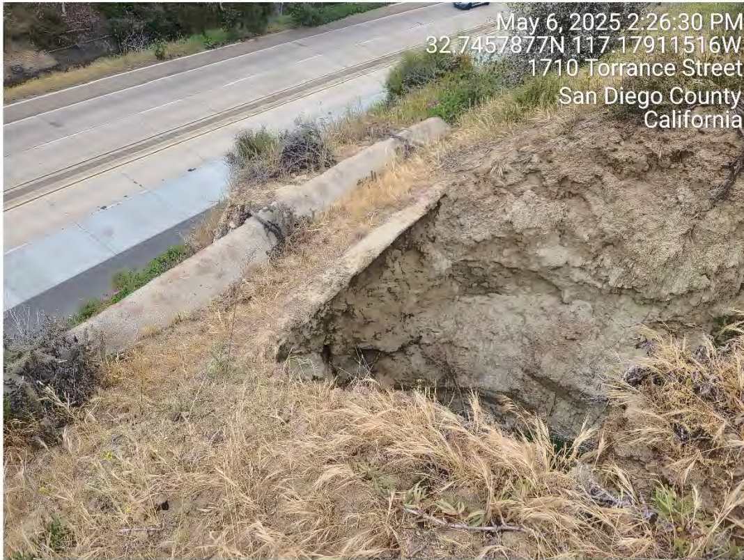
Sinkhole - view looking downstream at undermined brow ditch
