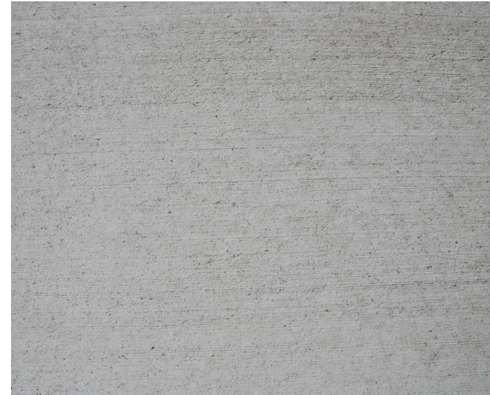
Standard Concrete Paving
